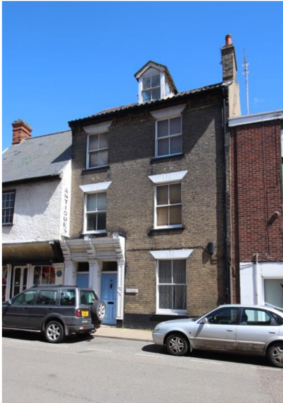
Suffolk white (or gault) brickwork
