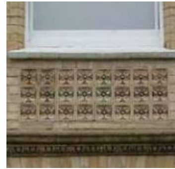
Moulded white brickwork, Station Road
