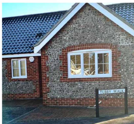
Combining materials - sandstone brick and flint
