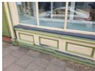
Example of panelled stallriser on traditional shopfront.
