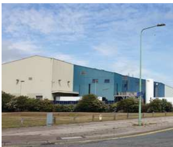
Graded colour corrugated steel on Birdseye Factory
