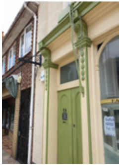
Traditional shopfront fanlight above front door, bounded by two wood pilasters.
