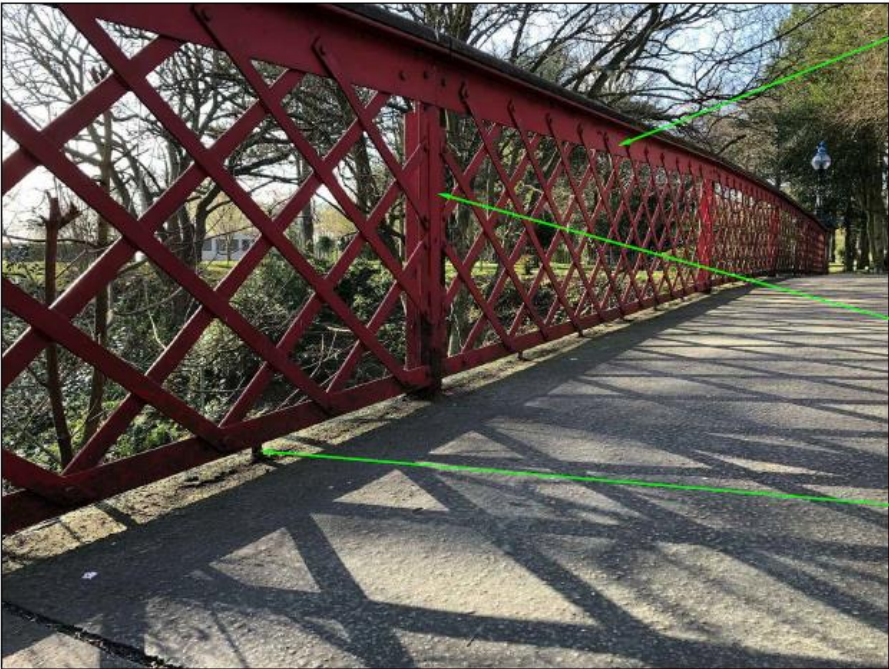
TYPICAL VIEW OF EXISTING NON-ORIGINAL FABRICATED MILD STEEL HAND RAIL INFILL PANELS & BALUSTERS
