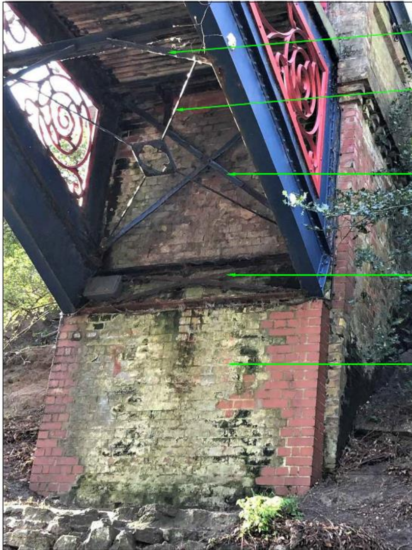
GENERAL VIEW OF SOUTHERN BRIDGE ABUTMENT SHOWING ARRANGEMENT OF WROUGHT IRON VERTICAL AND PLAN BRACING MEMBERS
