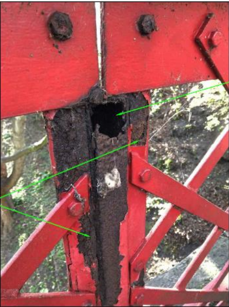
TYPICAL VIEWS SHOWING SEVERE LEVELS OF CORROSION AND SECTION LOSS PRESENT IN EXISTING FABRICATED MILD STEEL HAND RAIL BALUSTERS
