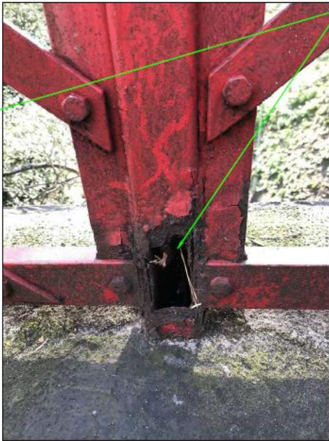
TYPICAL VIEWS SHOWING SEVERE LEVELS OF CORROSION AND SECTION LOSS PRESENT IN EXISTING FABRICATED MILD STEEL HAND RAIL BALUSTERS
