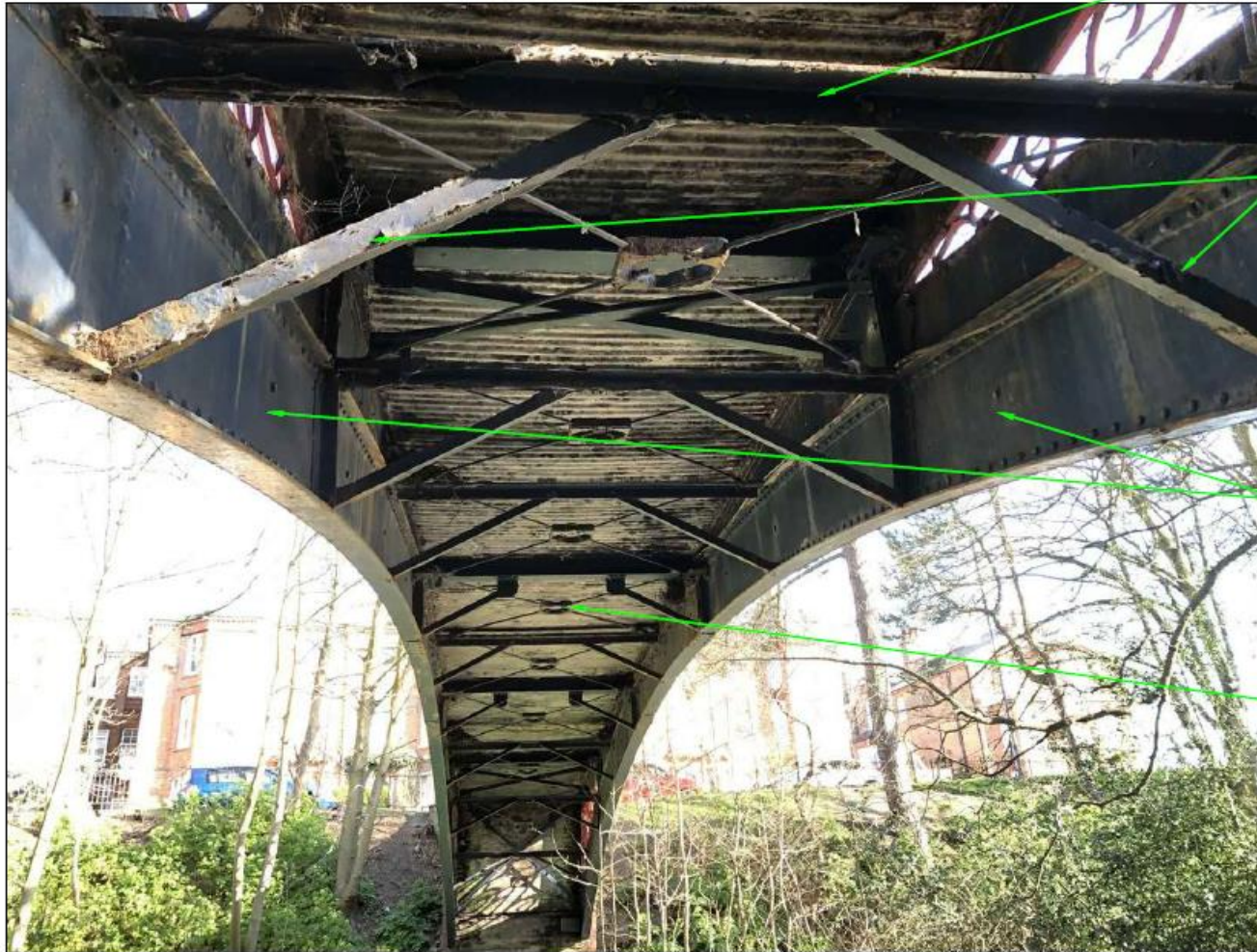
GENERAL VIEW OF UNDERSIDE OF BRIDGE DECK SHOWING PLAN BRACING MEMBER ARRANGEMENT AND BOTTOM FLANGE RESTRAINTS TO PRINCIPAL BRIDGE BEAMS
