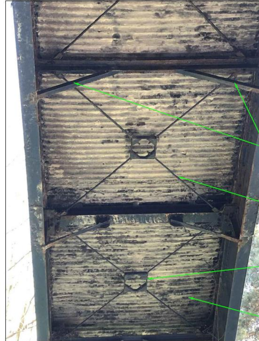
GENERAL VIEW OF UNDERSIDE OF BRIDGE DECK SHOWING PLAN BRACING MEMBER ARRANGEMENT
