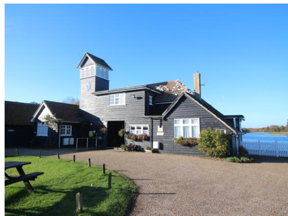
Black stained weatherboarding to the Boathouse, The Meare
