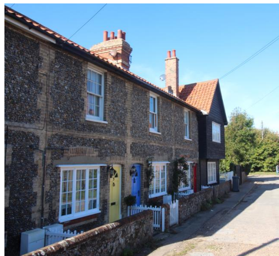
Washed cobble with white brick margins, Old Homes Road
