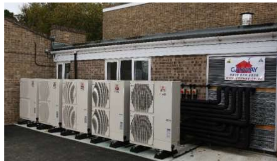
Figure 6 Air Source Heat Pump System
