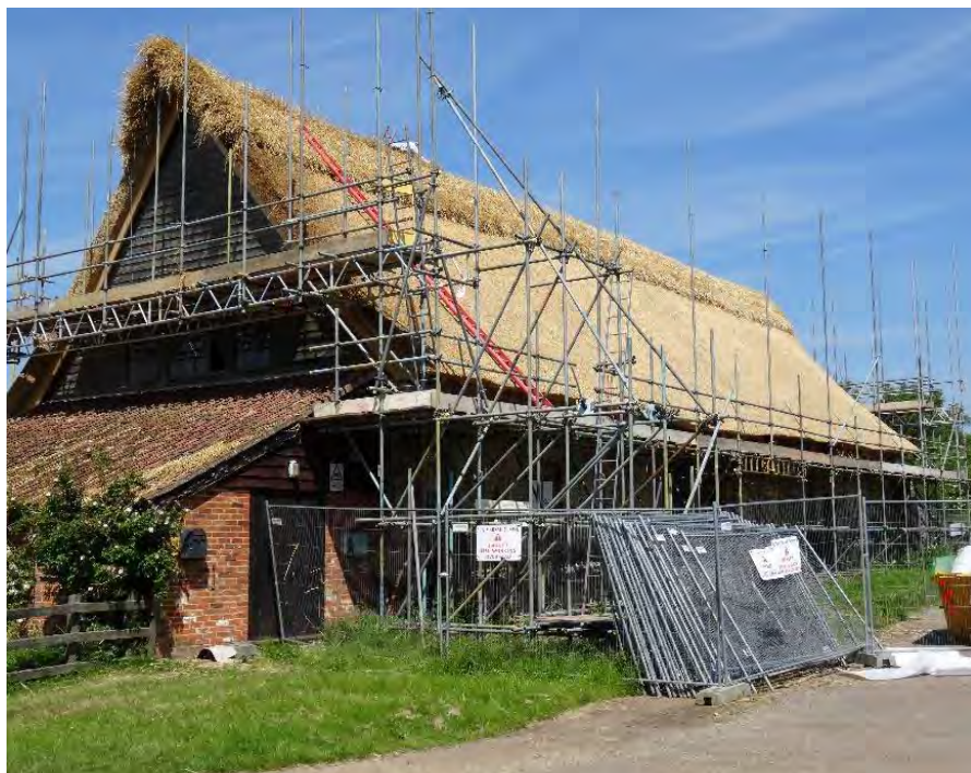
Replacement of thatch roof (Leiston Abbey Barn). (Source – Tim Buxbaum)
