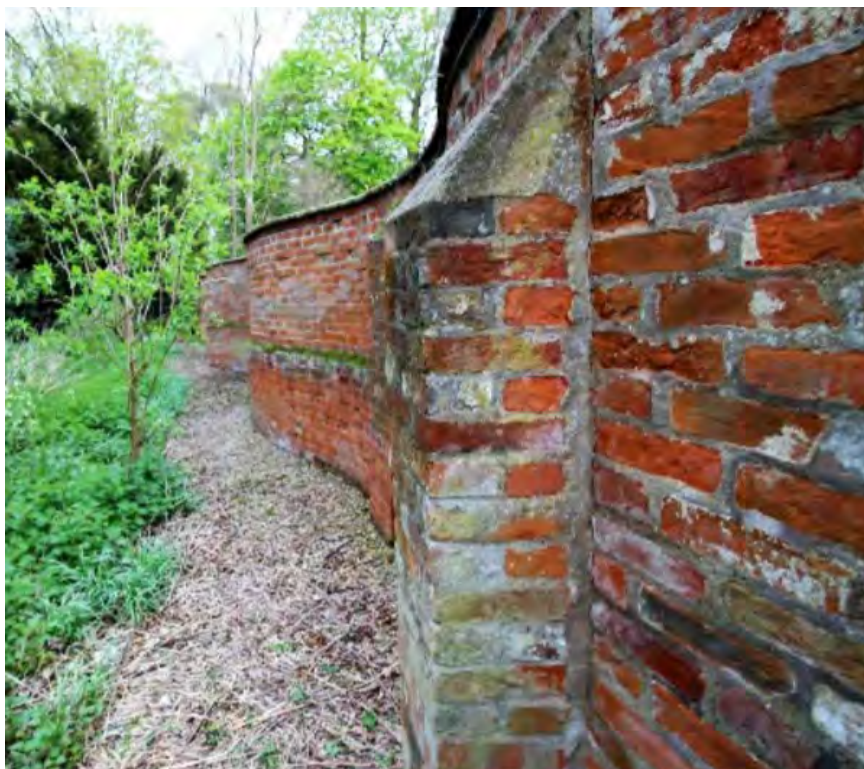
A crinkle crankle, or serpentine wall (Yoxford). (Source - Cockfield Hall Estate)
