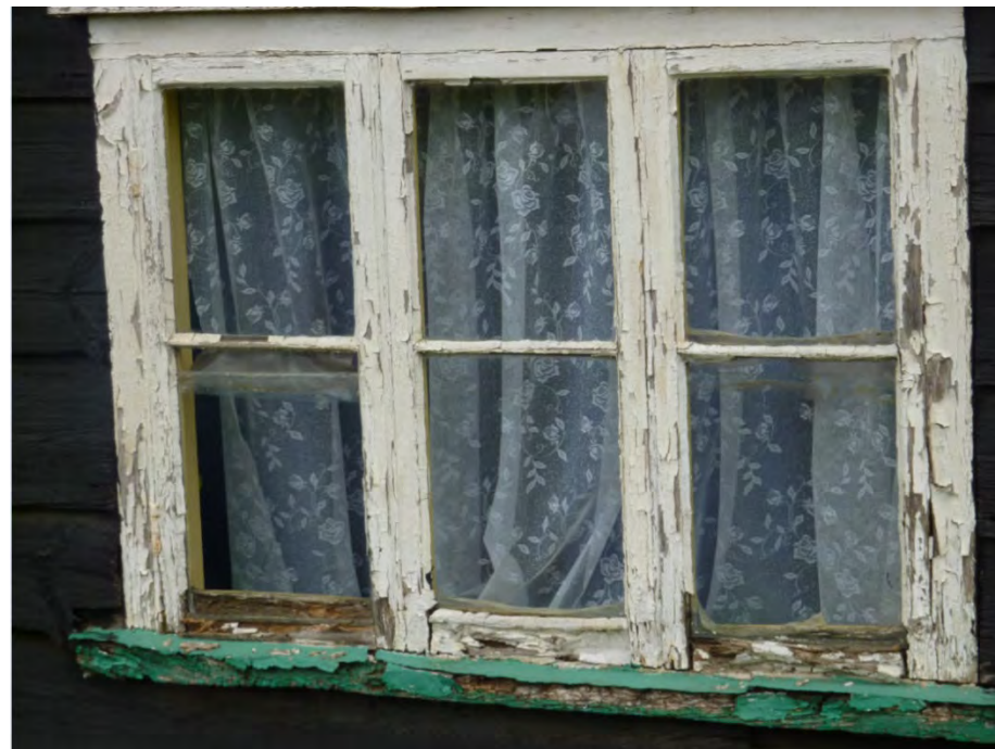
This window is in poor condition, but successful repair is possible.
