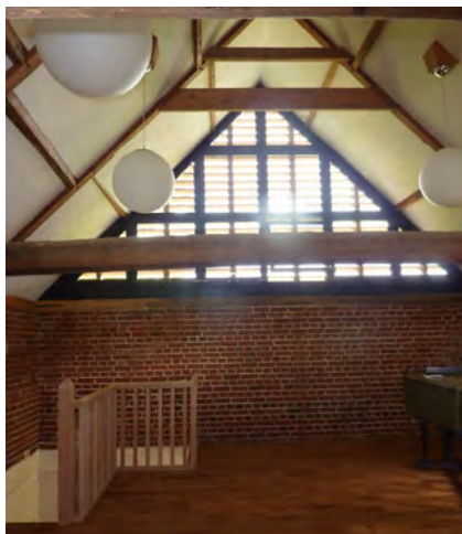
A new window that has been successfully inserted into the gable space of a barn, meaning no new windows inserted into the wall. Wooden slats reduce visual impact of the window (Hasketon Grange Barn) (Source – John Lamont)
