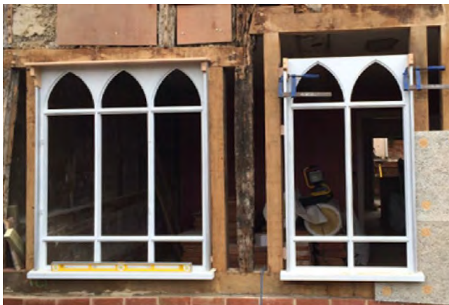
Traditional windows undergoing repair (The Agent's House, Easton). (Source – Roberts Molloy Associates)
