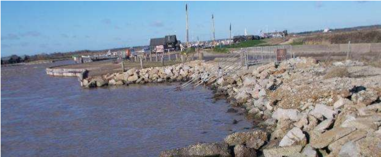
Figure 4-19: Rock revetment West of North Wall
