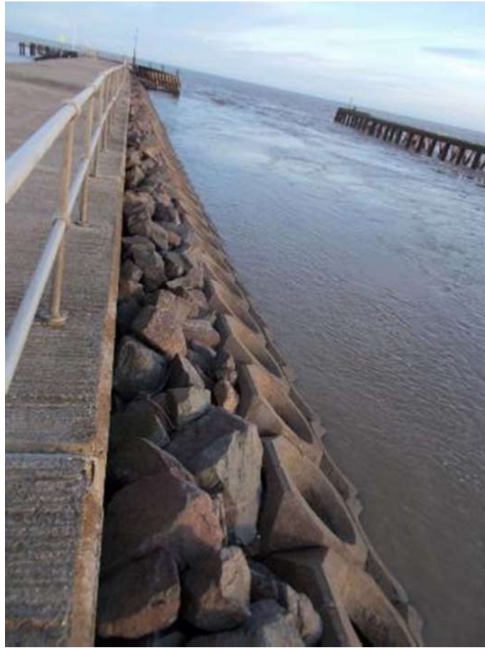
Figure 4-12: SHED concrete blocks with rock fill
