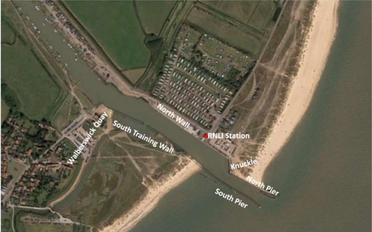
Figure 1-2: Southwold Harbour Structures
