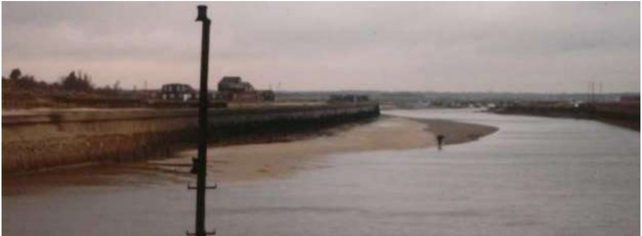
Figure 2-8: Sediment accumulation, south side of harbour, 1987
