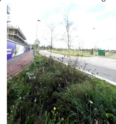
Planted buffer that contributes towards an attractive environment, management of surface water run-off, cooling, and enhanced safety through physical segregation between the cycle track/footpath and the carriageway. Waterbeach, Cambridge.
