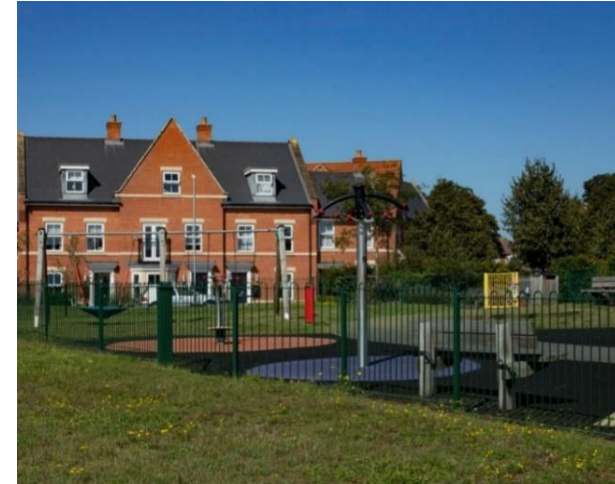
Fenced LEAP at The Sandlings, Martlesham – the fencing design is appropriate for its space setting.
