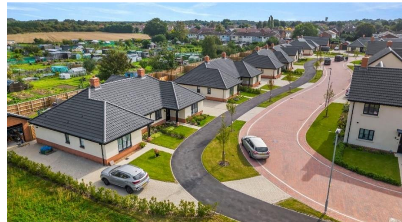
An accessible, segregated shared path supported by soft landscaped green buffer strips and tree plantings. The Lilacs, Trimley St Martin. Source: Aspen Build Ltd (www.aspenbuildltd.co.uk)
