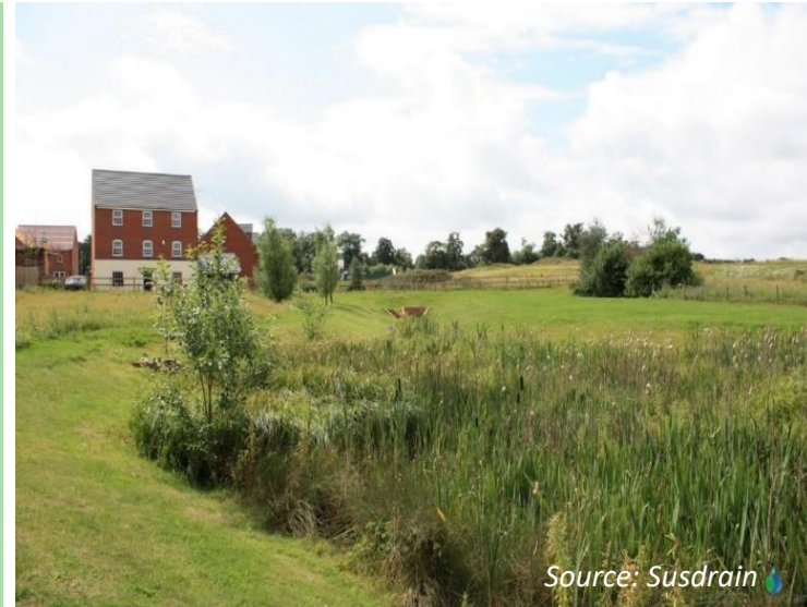
A nature-led sustainable drainage system (SuDS) scheme.
