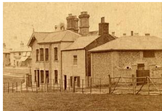
Historic view (undated), showing Gun Hill Cottage when in use as a stable and loft.
