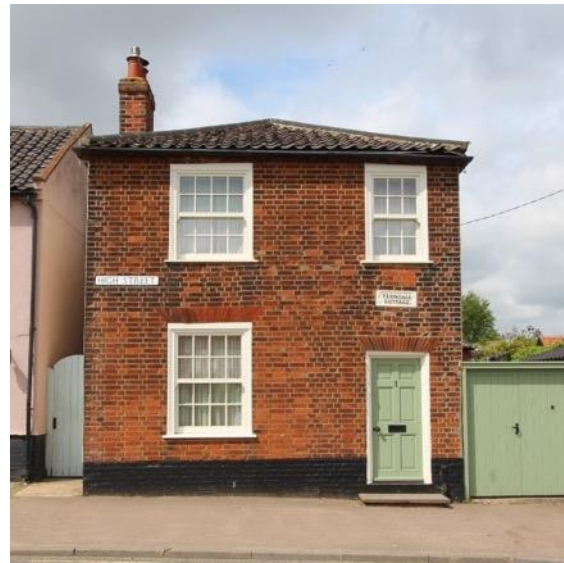
Ferndale Cottage, High Street
