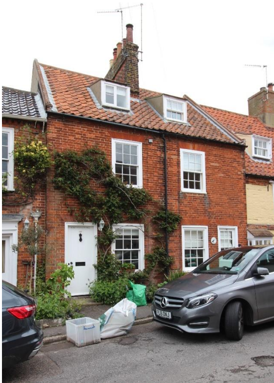
Nos.13 & 15 Park Lane
