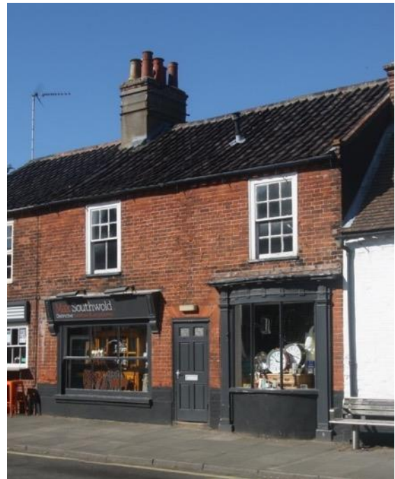
Early nineteenth century shop fascia at No.25 High Street.
