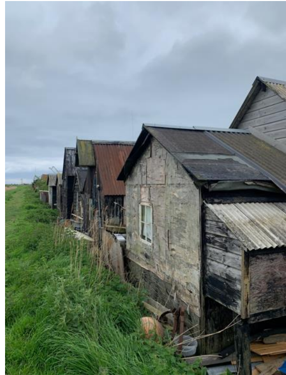
View of the rear elevation of huts, looking north east
