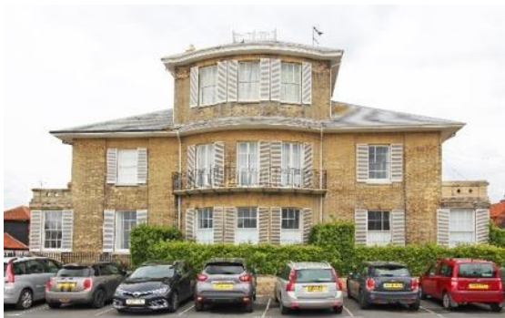
No.1 Greyfriars North, Greyfriars South, and Regency House, South Green
