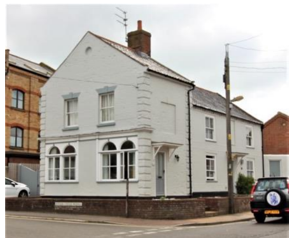
No.2 High Street, Field Stile Road elevation
