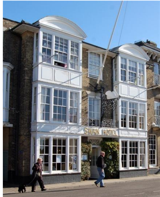
The Swan Hotel, Market Place, a c.1907 reworking of an early nineteenth century façade for Adnams.
