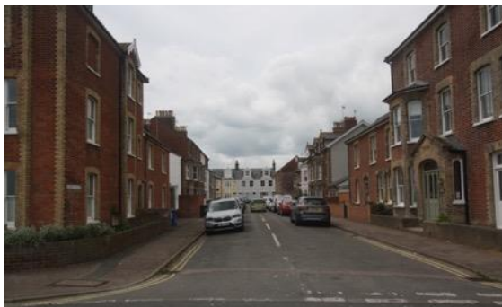
Chester Road / North Parade: loss of historic boundary treatments.
