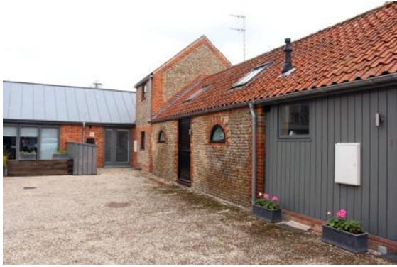
Snowdens Yard: rooflights set into traditional roof materials.
