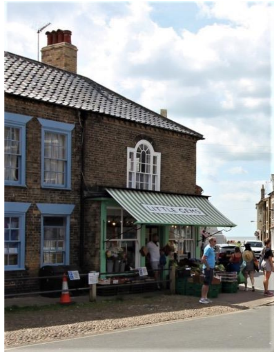
No.21 Market Place with mid to late nineteenth century wide sashes to its fascia associated with food retail.
