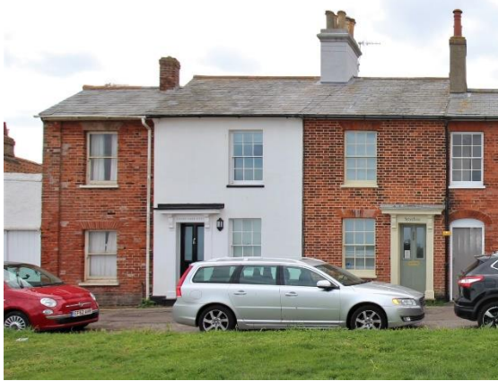
Nos.7 & 8 East Cliff showing late twentieth century addition to left.
