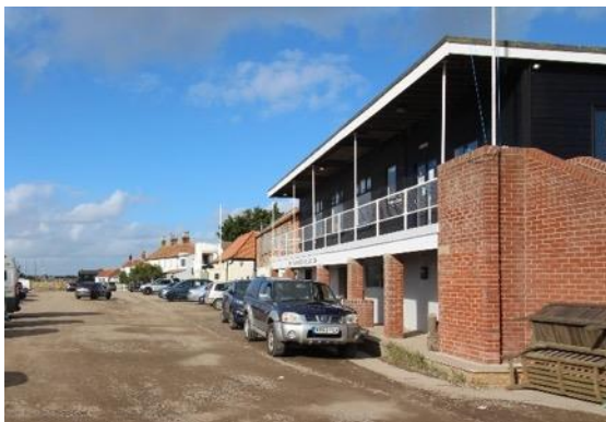
The Sailing Club Building, Blackshore Quay
