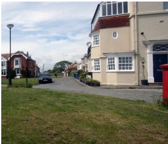
Granite Setts outside No. 2 Park Lane
