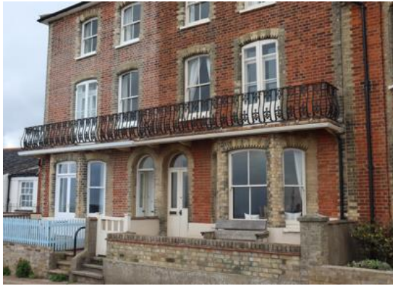
Elegant railings to first floor balcony, North Parade.
