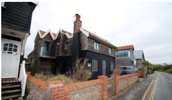
Ferry Road: the rebuilding of 20th century ribbon development retains some of the idiosyncrasies of the earlier structures but with greater formalisation of boundaries, modern building materials and more ambitious scale, incrementally changing the road's modest 20th century character.
