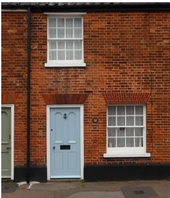
View of 8 over 8 pane hornless sash windows.
