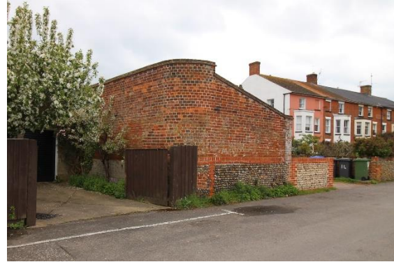
Wall enclosing courtyard at The Anchorage, No.14 Cumberland Road
