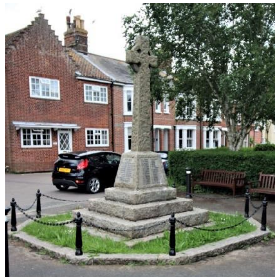
War memorial with well-made bitumen macadam surfacing and large pitted granite kerbs, although the chain and bollards lack any local distinctiveness.
