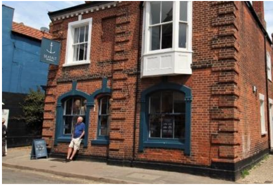
The c.1856 frontage of the former Victoria Public House on East Street survives remarkably intact.
