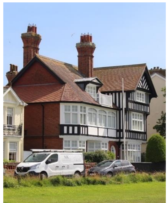
Half-timbering and 'jettied' accommodation to a late 19th / early 20th century villa on Godyll Road.
