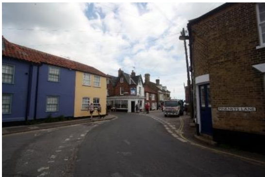
Pinkneys Lane: strong enclosure created by the sinuous street layout and buildings that tightly control views.
