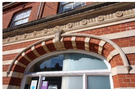
Detail of No.67 High Street.
