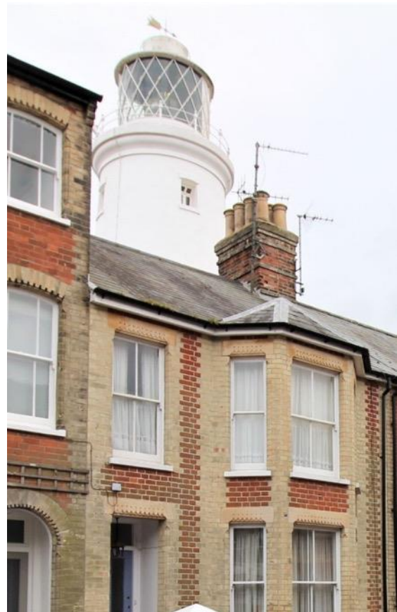
Chester Road: recently cleaned brick work.
