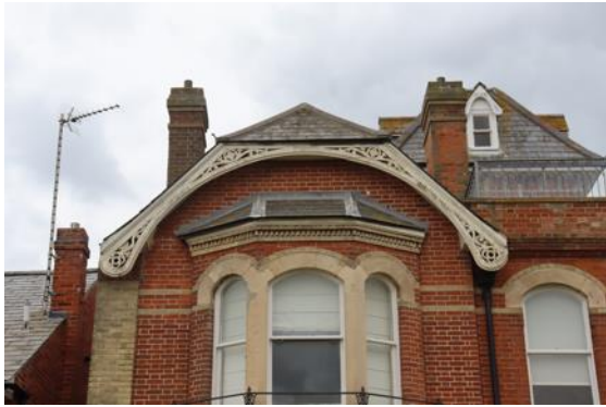
Slate roof covering.
