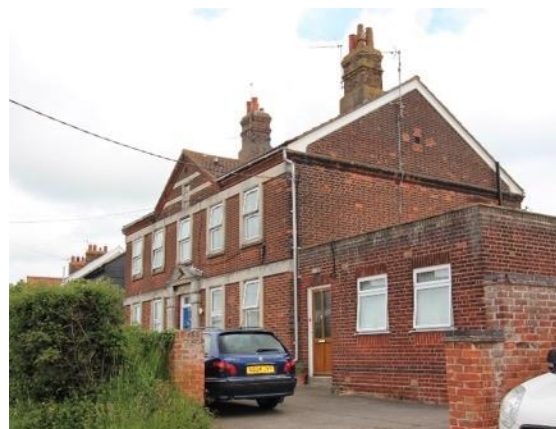
Nos. 21-27, Station Road
