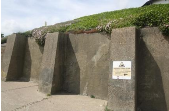
Sea Aster softening the top of the cliff revetments.
