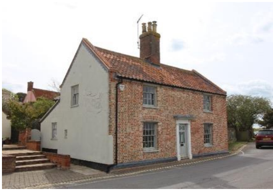
Saltworks Cottage, No.6 Ferry Road
