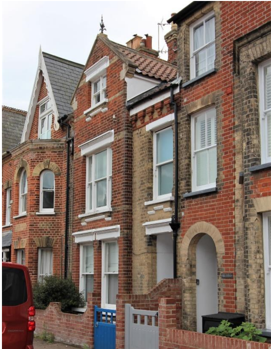
No.50 Stradbroke Road
