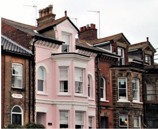
Chester Road: Colour washes can result in a unified terrace's visual 'rhythm' being disrupted and the masking of gault brick dressings.
