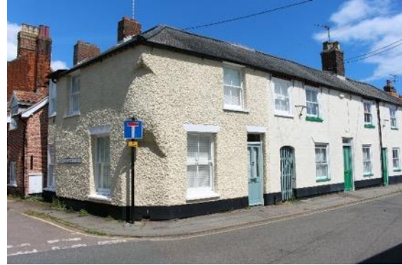
Nos.12-18 (even) Victoria Street, from Bartholomew Green: street signage clutters and obscures the architectural detailing.
