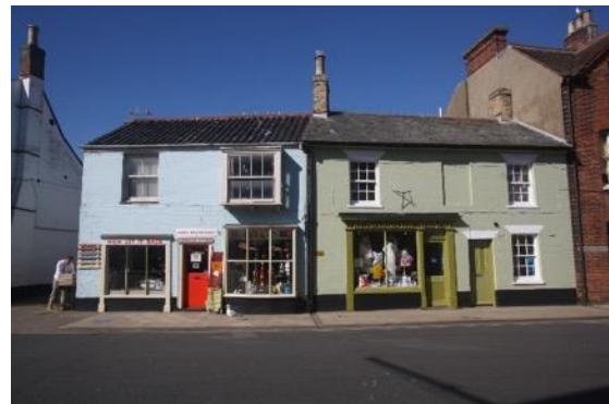
Colour washed brick (left) and render (right), using modern colour palettes. Colour washing and renders have become part of the Old Town's retail character, such as on the High Street.
