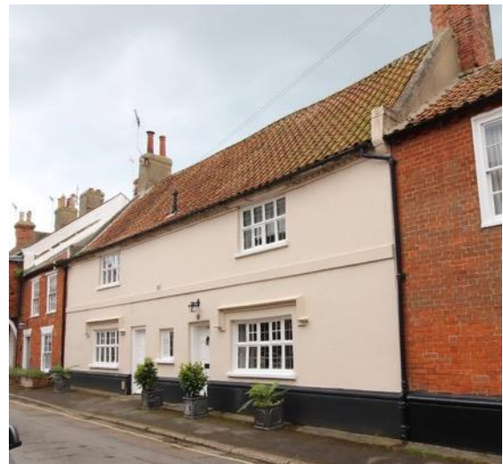
Nos.16 & 18, Park Lane
