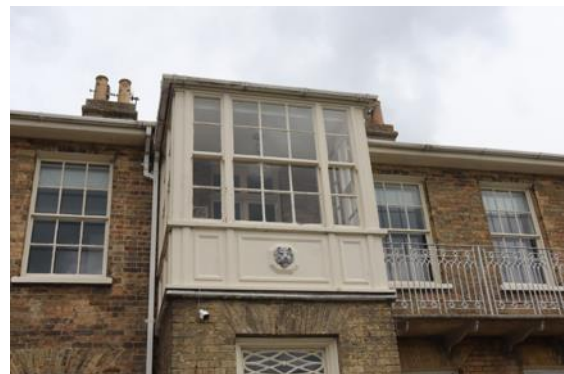
Timber square bay window.
