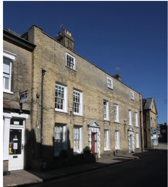
No.1 The Elms and No.3 Queen Street
