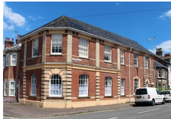
Chester Road: Modern, altered, façade of a former shop that presents a strong corner accent with decorative quoins, dressings and pilasters with gault brick.
