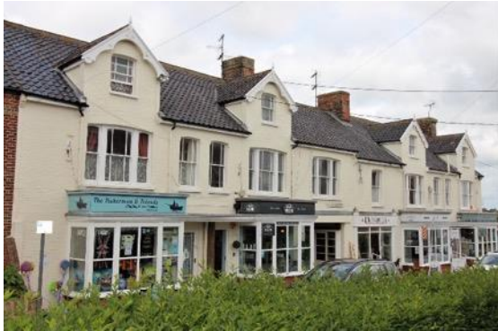
Nos.3A-9A (Odd), Station Road
