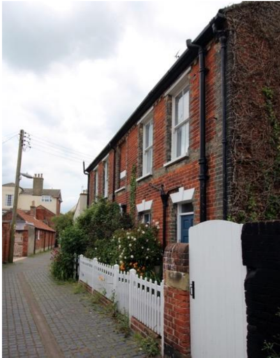
Bank Alley: Staffordshire Blue cubes / setts, laid in rows around a concrete drainage gully. Hard wearing floorscape materials, such as Staffordshire Blue cubes / setts, positively contribute to the character of the Conservation Area and identify the street as a route being used for heavier traffic, with an important connection to the church.
