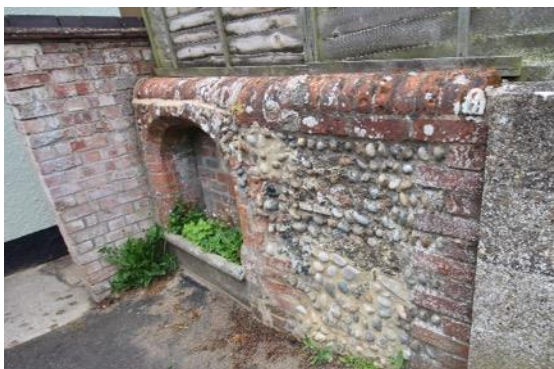
Water trough on Ferry Road positively contributes to the historic environment.
