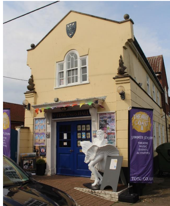
Southwold Arts Centre, Cumberland Road
