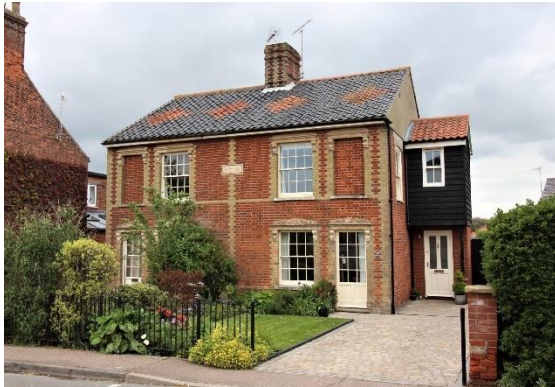
Victoria Cottages, Nos.24 & 25 Field Stile Road
