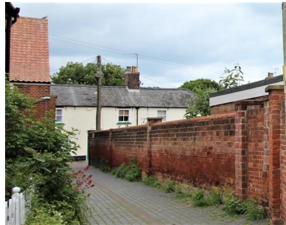
Electricity Substation Boundary Wall, Bank Alley
