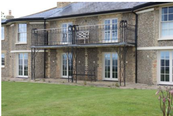
Restrained iron railings, supported below to form first floor balcony and covered ground floor veranda
