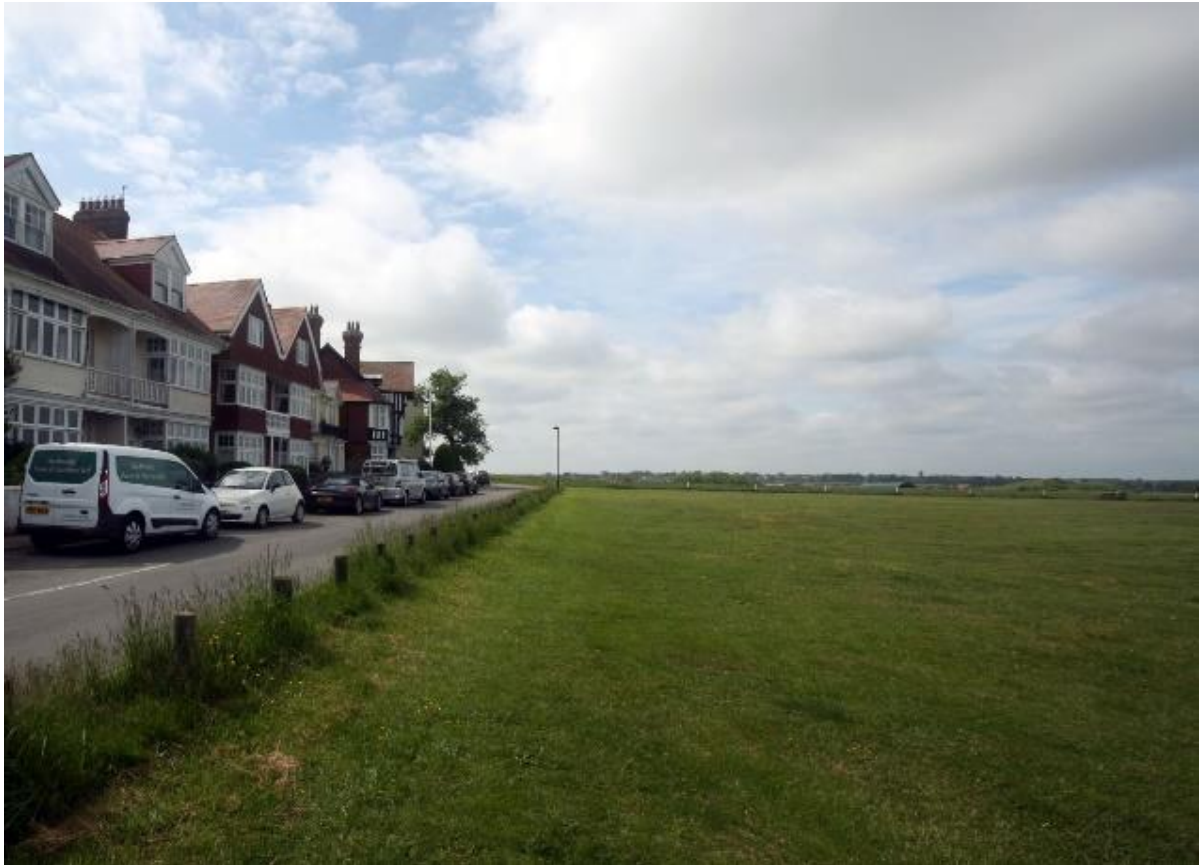
View of dwellings on Godyll Road, designed to maximise landscape and sea views.
