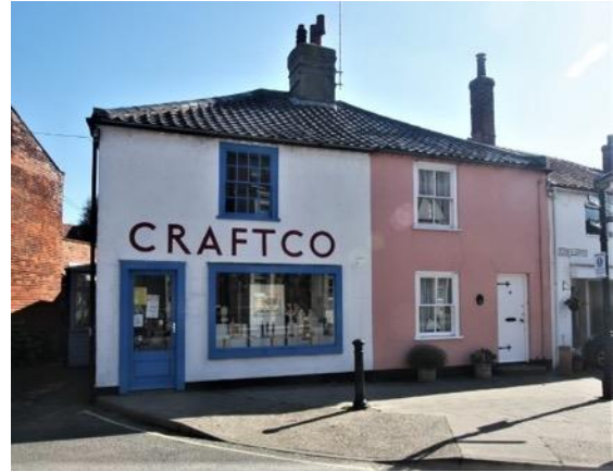
Unsympathetic shop window at No.40A High Street.
