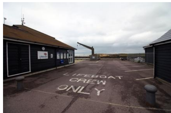
Features such as the winch at Southwold Harbour for use by the RNLI adds interest to a sparsely used area and further highlights the site's use with activity specific infrastructure.
