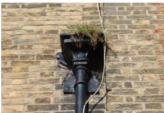
Detail of an early 19 th century rainwater hopper.
