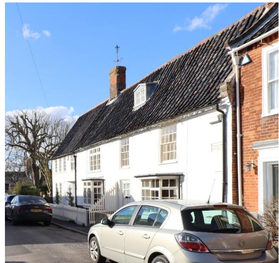
Nos.21 & 23 Park Lane
