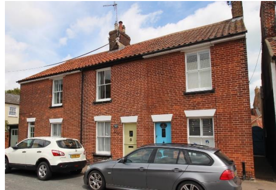
Palm Cottage, No.34 & 34A Victoria Street
