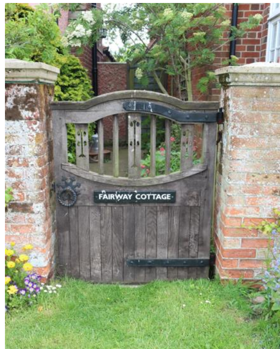
Timber hand gate with bespoke strap hinges and ring handle, designed to complement the timber screen.
