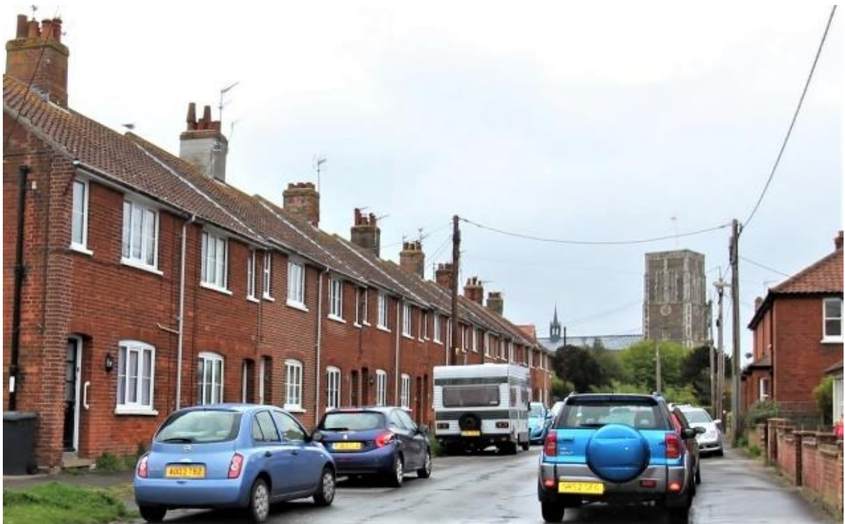
The parish church from St Edmunds Road and early council houses of c.1905
