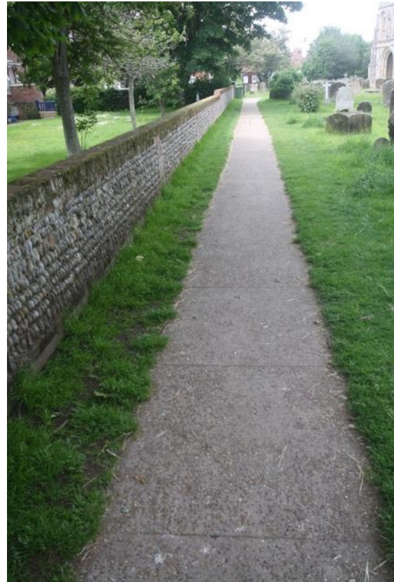
Exposed aggregate, in situ, concrete path within the churchyard of St Edmund the King and Martyr's Church. Whilst the material has little in keeping with the churchyard environment is likely a local aggregate and has association with the seascape environment.
