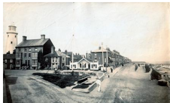
St James' Green: prior to cement render on earlier block wall and steps.
