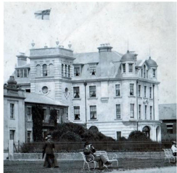
George Skipper's bedroom wing to The Centre Cliff Hotel of c.1905, its two upper floors have since sadly been removed.
