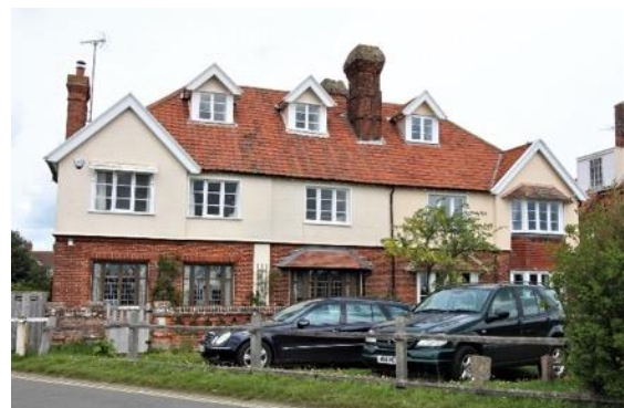
No.5 (right) and No.6 (left) and boundary wall, Strickland Place
