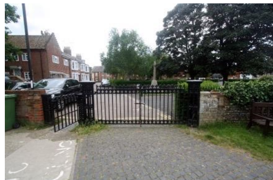
Staffordshire Blue setts / cubes within the churchyard of St Edmund the King and Martyr's Church, adjacent to the public space's principle entrance, is juxtaposed with the Regency Gothic cast iron churchyard gate of 1838. The use of a robust material denotes the route's importance for ceremony and vehicle access.
