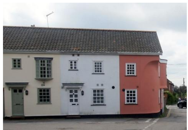
14 Mill Lane: strong corner to the street junction.
