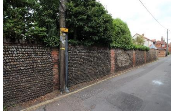
Boundary Wall to No.7 Mill Lane
