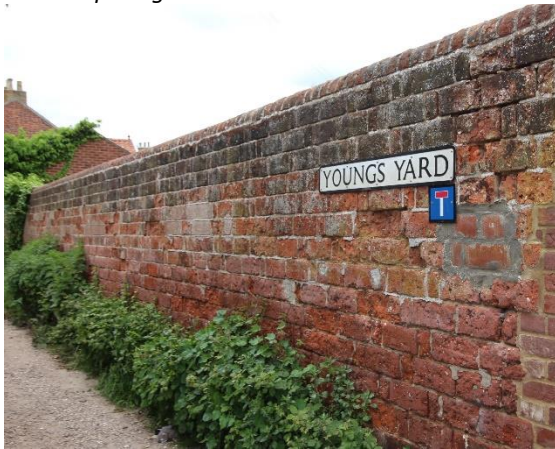
Boundary Wall to Electricity Substation on Northern Side of Youngs Yard
