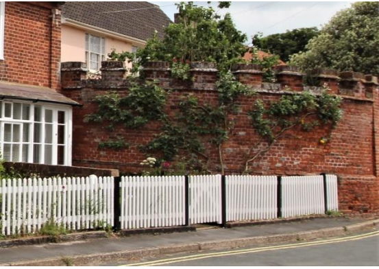
Western Section of Garden Wall to No.9B Lorne Road
