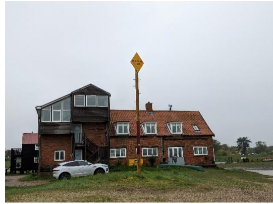
Figure 30 The Old Yacht Yard (Boat House) from the east, showing modern alterations
