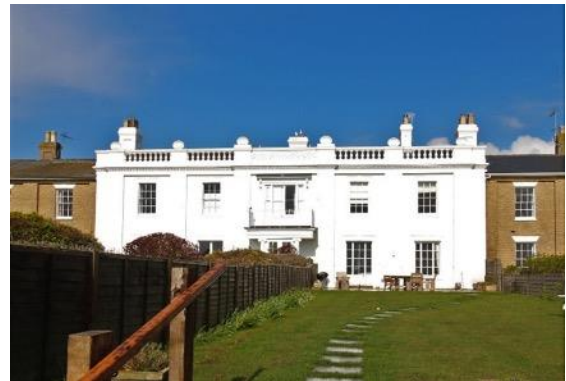
Nos.1 & 2, Centre Cliff, South Green
