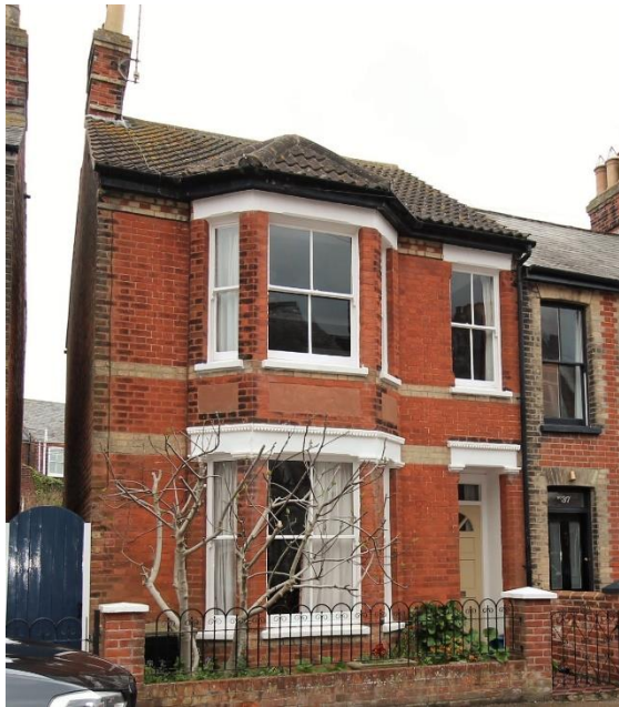
No.39 Stradbroke Road
