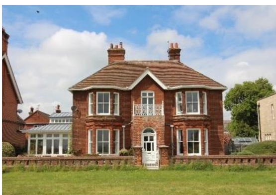
Wantage House, gate and boundary wall, The Common
