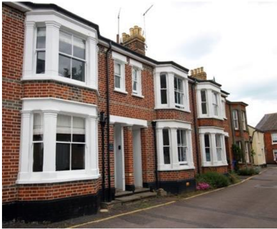
Typical Southwold townscape detail, with the buildings hard to the highway edge.
