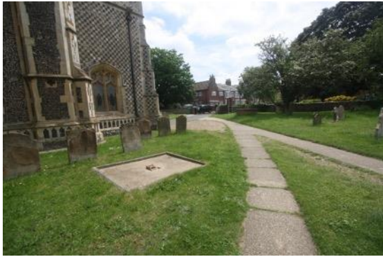
Concrete pad (likely the base for a now removed bench) and white paint signs are not in keeping with the churchyard's character.
