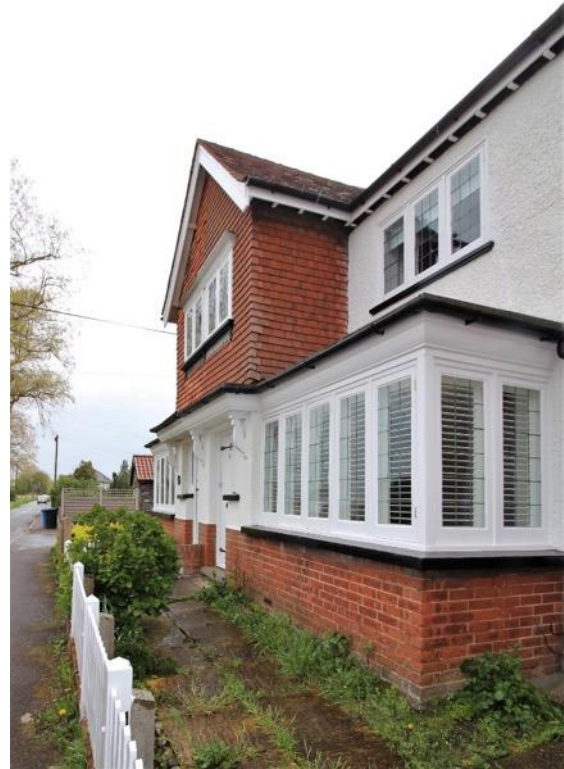
Nos.27 & 29 North Road
