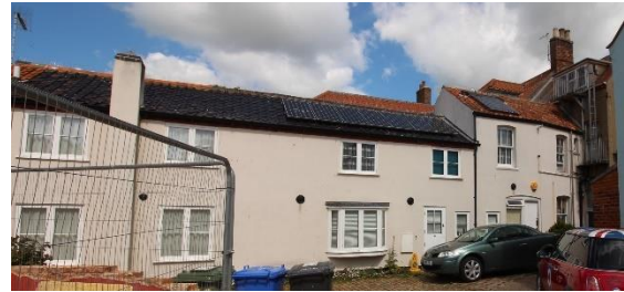
Rear of No.1 and Nos.7A & B Market Place
