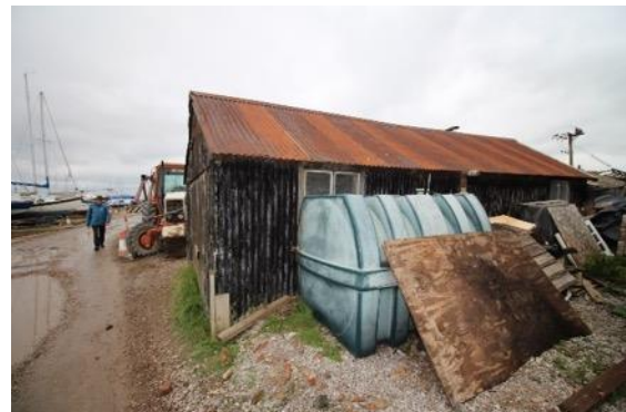
Part of Justin Ladd's Boat Building sheds
