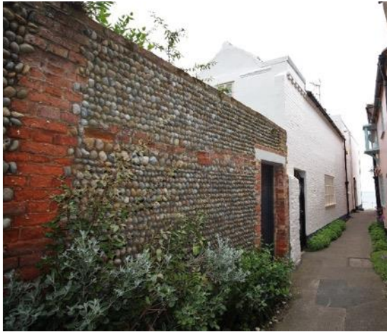
Boundary wall, to the west of The Nook, Primrose Alley
