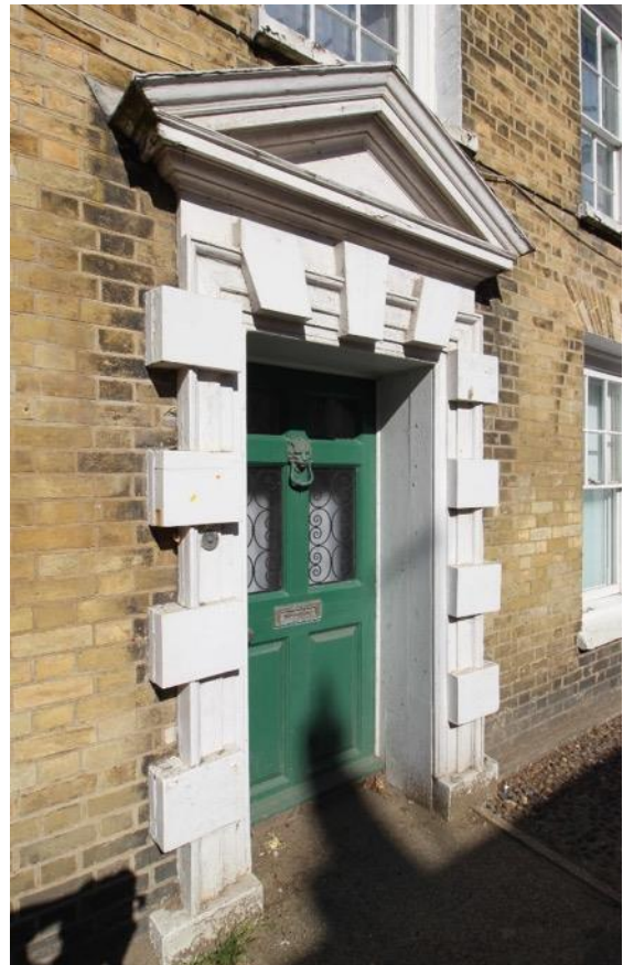
One of a pair of Gibbsian Doorcases at Nos. 1 & 3 Queen Street. The right hand doorcase is of mid to late eighteenth century date whilst that to the left-hand house dates from c.1925.
