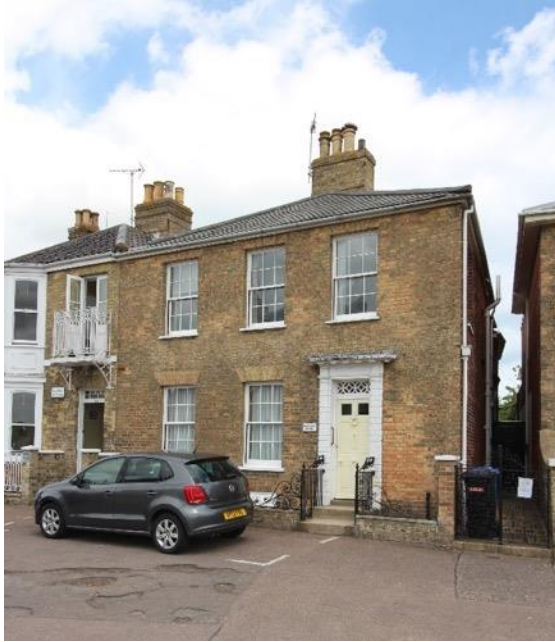
South Green Cottage, No.6 South Green
