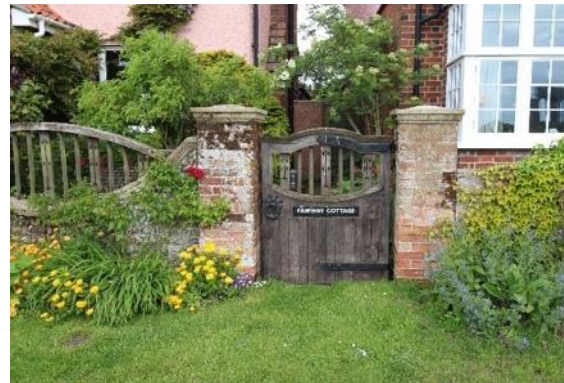
Timber hand gate, Fairway Cottage, The Common
