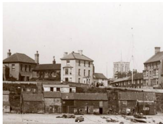
Nos.19 and 20 East Cliff, and No.21 St James Green c.1880
