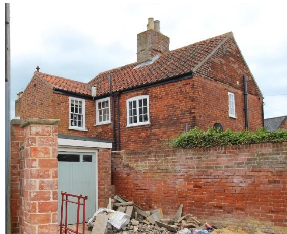
Nos.1 & 2 Youngs Yard from Bank Alley
