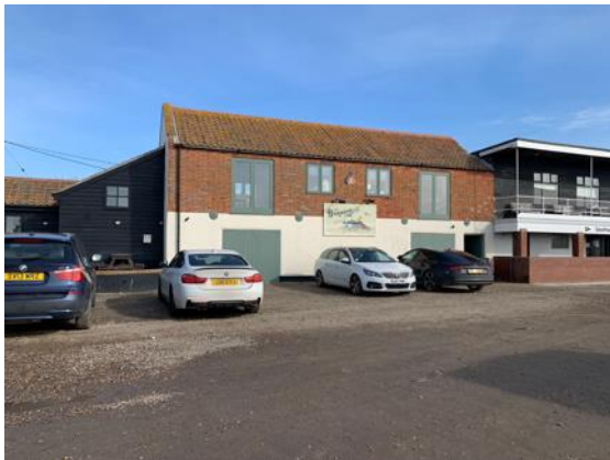
Former Warehouse, The Harbour Inn, Blackshore
