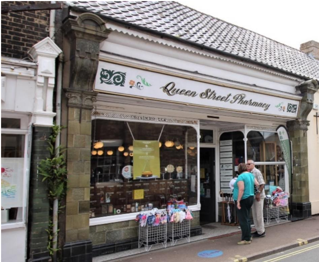
The former International Stores, No.18 Queen Street, a fine early twentieth century shop front of tile and cast iron.
