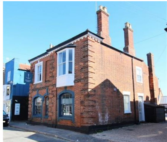
No.8 East Street: An externally well-preserved former public house that is now a shop.
