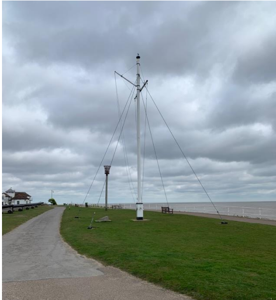
Timber mast, Gun Hill
