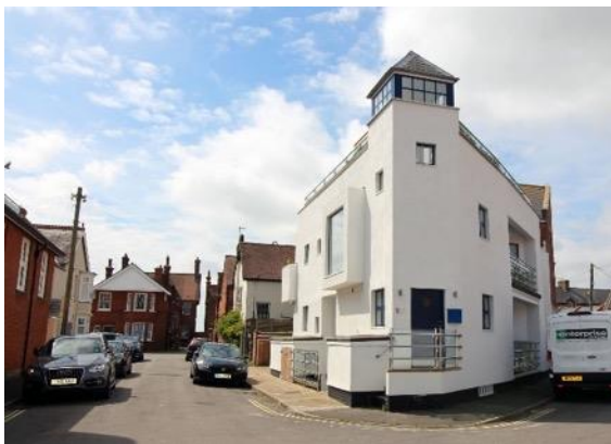
Blackmill Road: Contemporary 'infill' development on the former Southwold and Reydon Royal British Legion site presents a notable departure from its built form context.
