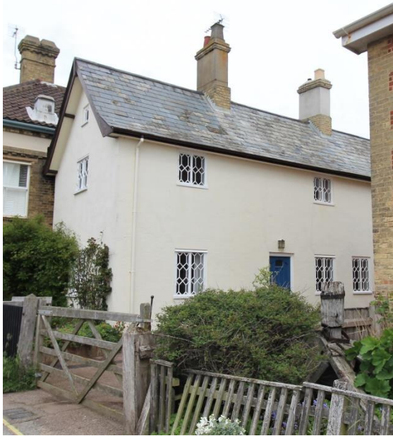
Reading Room Cottage, East Street
