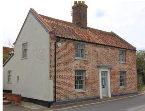
Ferry Road: Pargeting to the side of the building, visible from the public carriageway.
