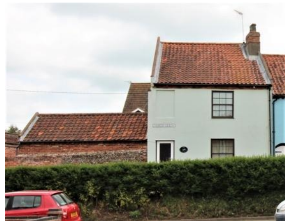
No.1 North Green and boundary wall
