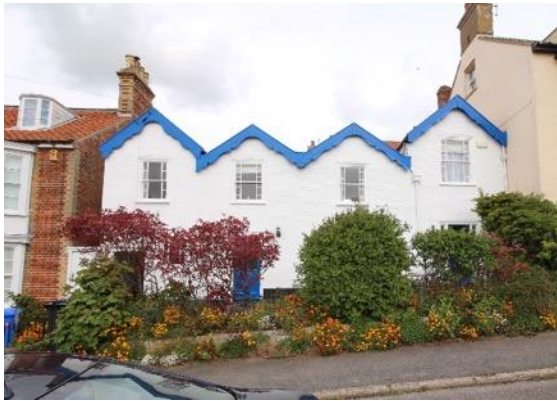
Iona Cottage No.11 and Iona Flat, No.11A Constitution Hill
