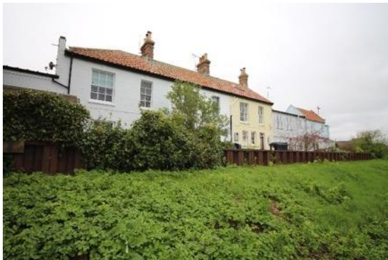
Rear elevation of Blackshore Cottages from the footpath
