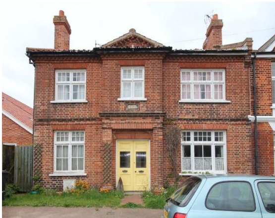
No.1 Cautley Road
