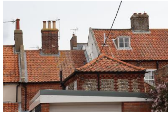
Red clay pan tile roof covering.
