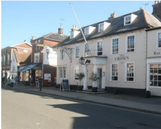
Hanging sign at The Crown, High Street
