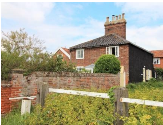
Spinners Cottage, west elevation and boundary wall, Spinners Lane
