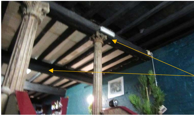
The partial replacement of the stud walls will be under these two existing beams. The pillars are temporary and only decorative.
