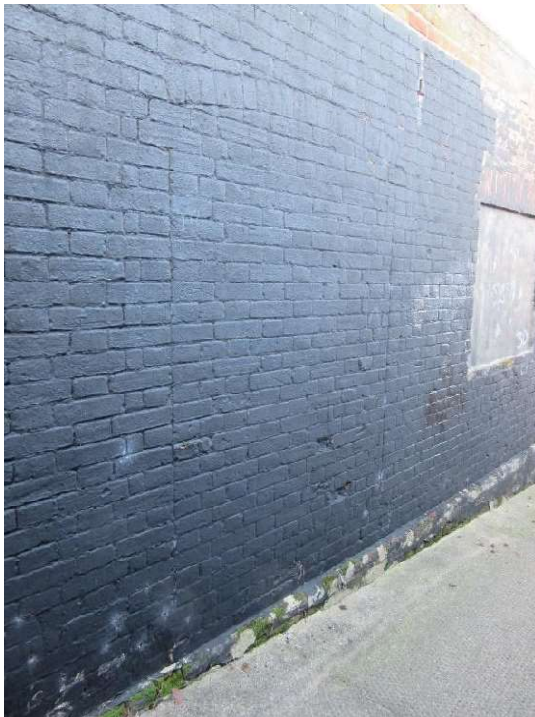
Proposed position for entrance doors to storage area. Evidence of a former opening here.
