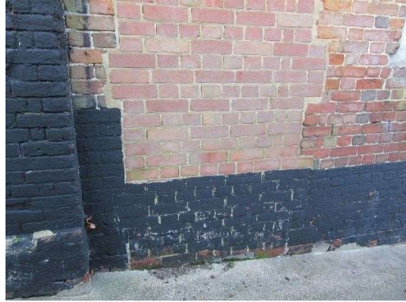
Proposed position for entrance door to warehouse. Evidence of a former opening here.
