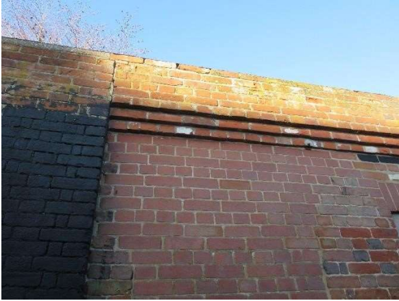
Proposed position for entrance door to warehouse. Evidence of a former opening here.
