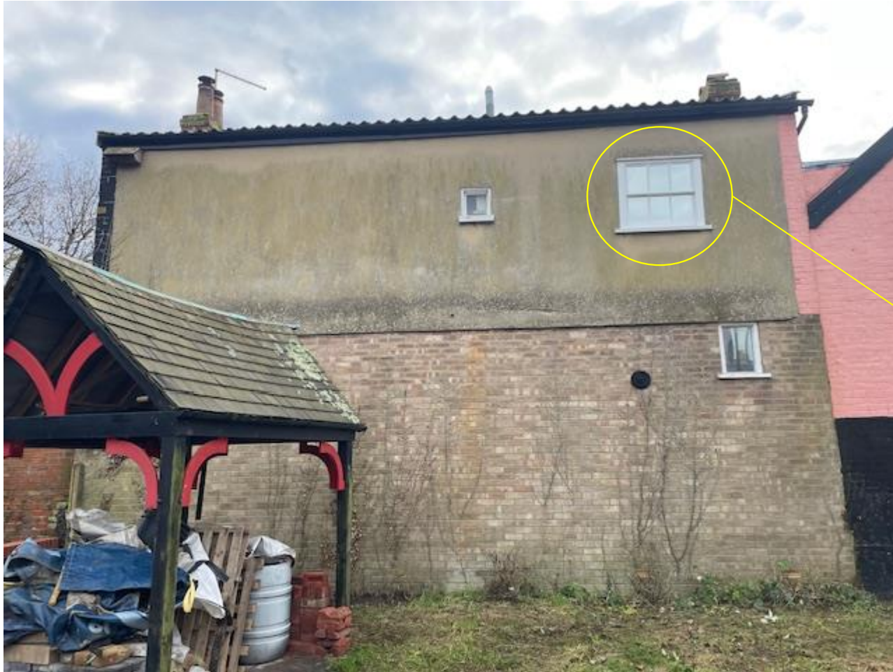
Officer photo of side elevation of 6 Doric Place from within site
