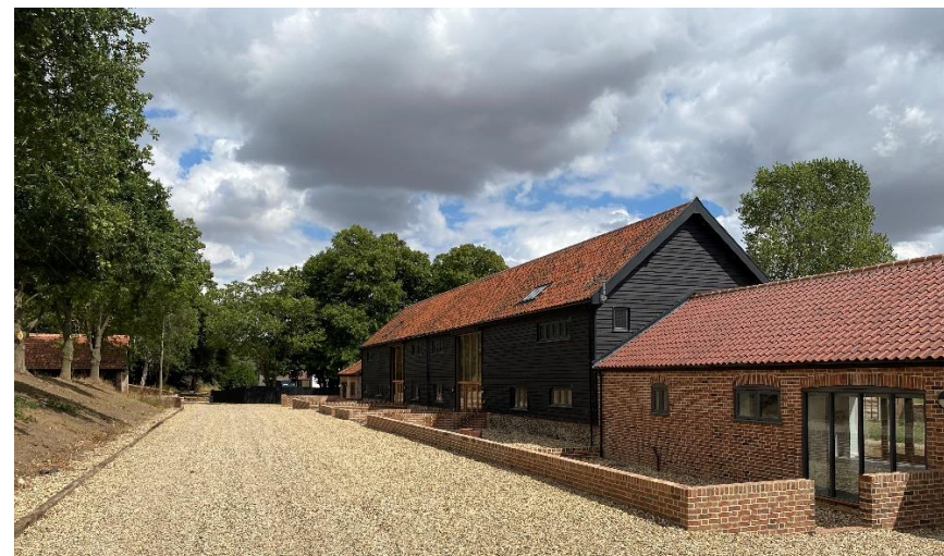
Converted agricultural buildings (Source: Clive Tanner FRICS, Hollins Architects, Surveyors & Planning Consultants)
