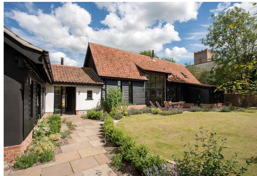
A well-designed barn conversion with the agricultural character retained, Church Farm Barn, Thorndon (Source: Craig Beech, Beech Architects)
