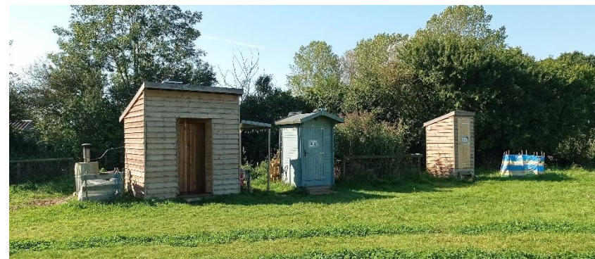
Associated toilet and shower block, Church Farm Glamping and Campsite, Redisham
