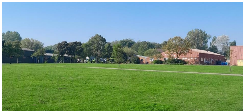
Buildings at Otley College blend into the landscape
