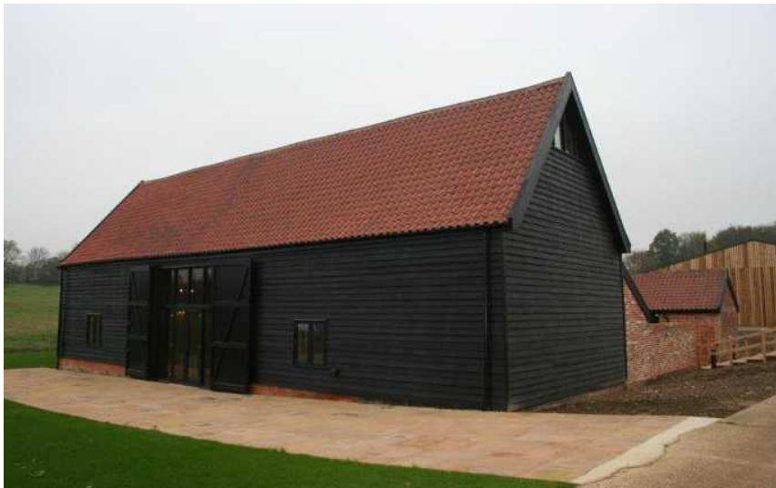
Barn converted with unbroken roof expanse retained, Bruisyard Hall Barns wedding venue (Source: Clive Tanner FRICS, Hollins Architects, Surveyors & Planning Consultants)
