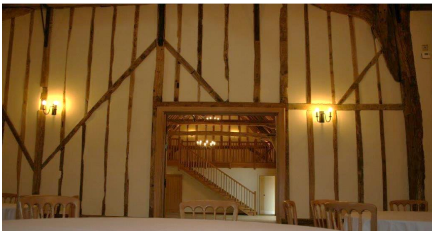
Converted barn with exposed timber stud walls retained, Bruisyard Hall Barns wedding venue (Source: Clive Tanner FRICS, Hollins Architects, Surveyors & Planning consultants)
