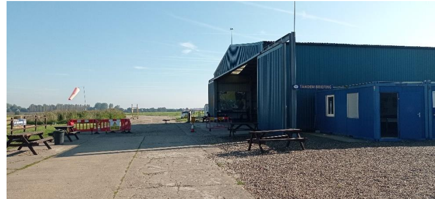
Hangar at Beccles airfield
