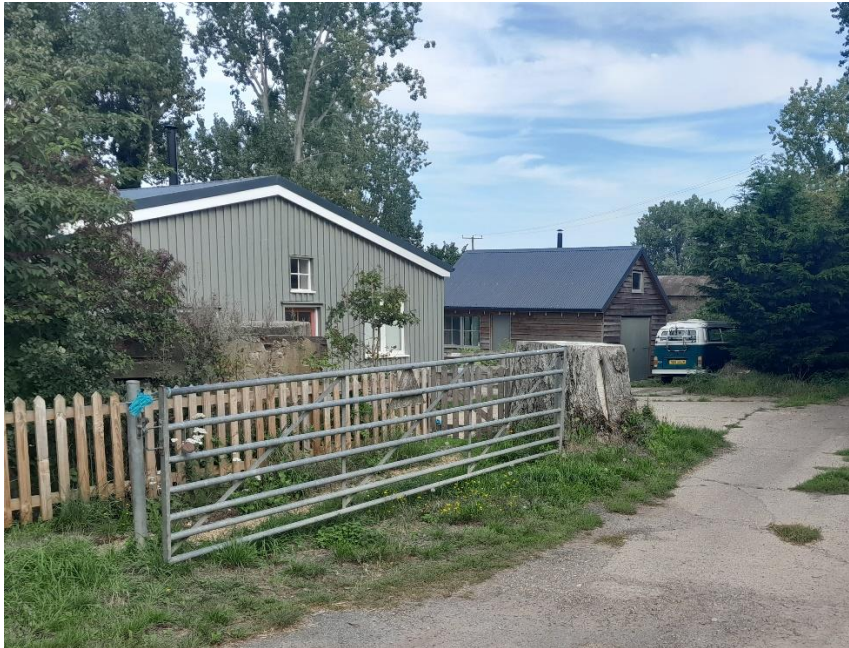
Agricultural building converted Under Class Q Permitted Development Rights, Mells, Halesworth
