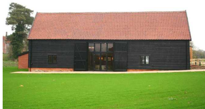
Converted barn with a limited number of openings in the wall, Bruisyard Hall Barns wedding venue (Source: Clive Tanner FRICS, Hollins Architects, Surveyors & Planning Consultants)
