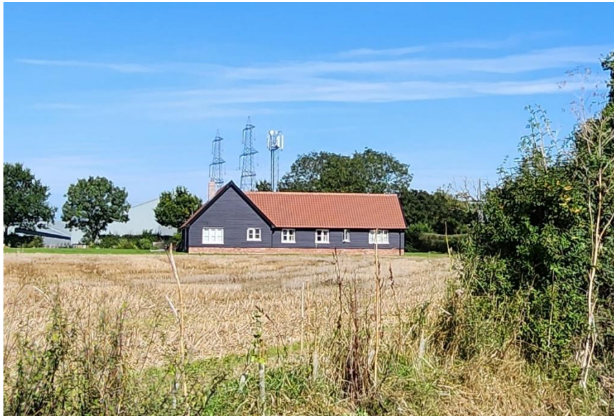
Rural workers dwelling
