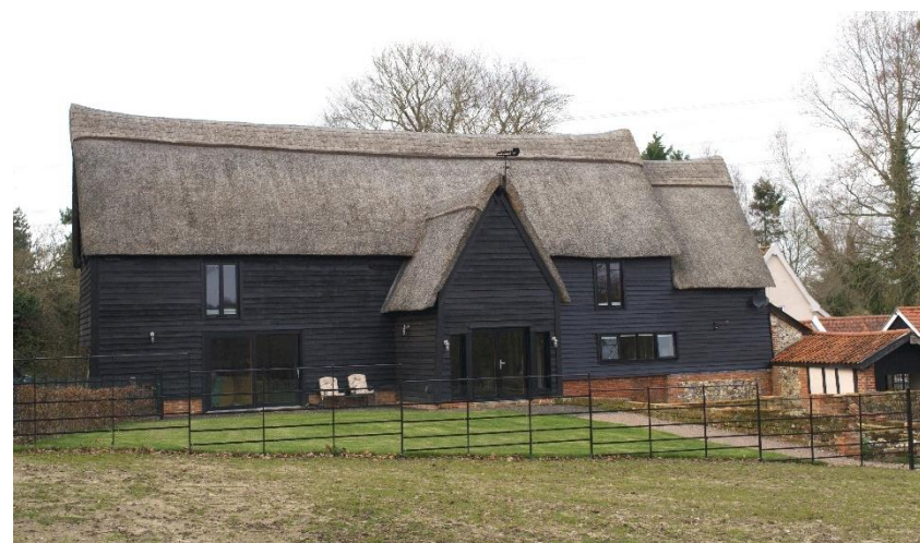
Llama Barn (Source: Mullins Dowse Architects)
