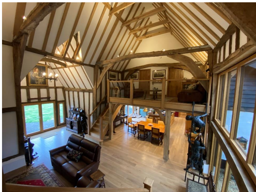
Llama Barn (Source: Mullins Dowse Architects)
