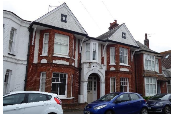
Figure 42 No. 6 Park Lane
