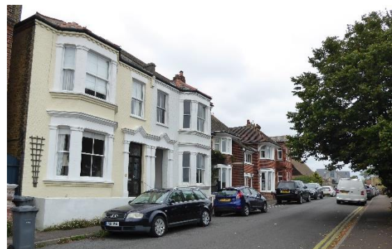
Figure 26 Nos. 21 - 23 The Terrace
