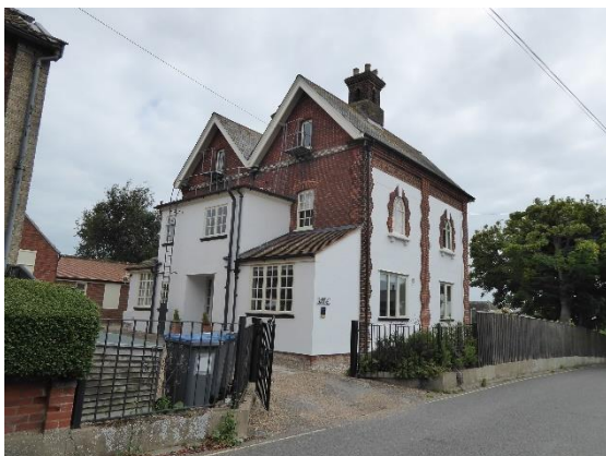
Figure 59 The Gables, Lee Road elevation
