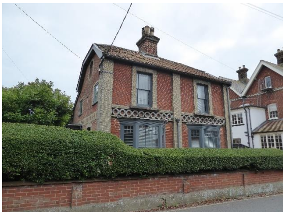
Figure 56 No. 8 Crespigny Road
