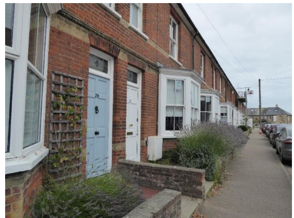
Figure 23 Terraced housing on Park Lane
