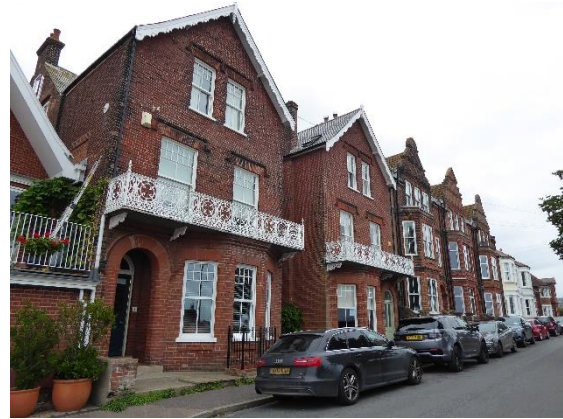
Figure 28 Nos. 31 - 33 The Terrace
