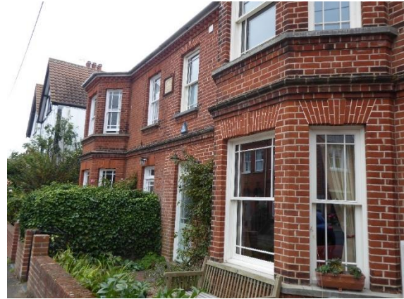
Figure 22 Example of red brick villa with bays, sashed windows, decorative banding, and dog toothed eaves detailing
