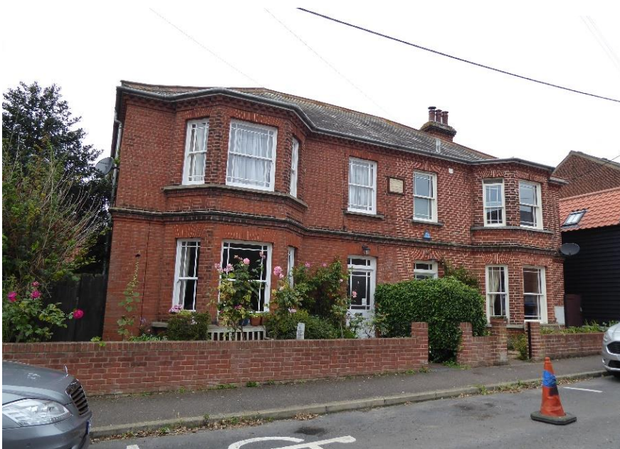
Figure 13 Villa on Fawcett Road
