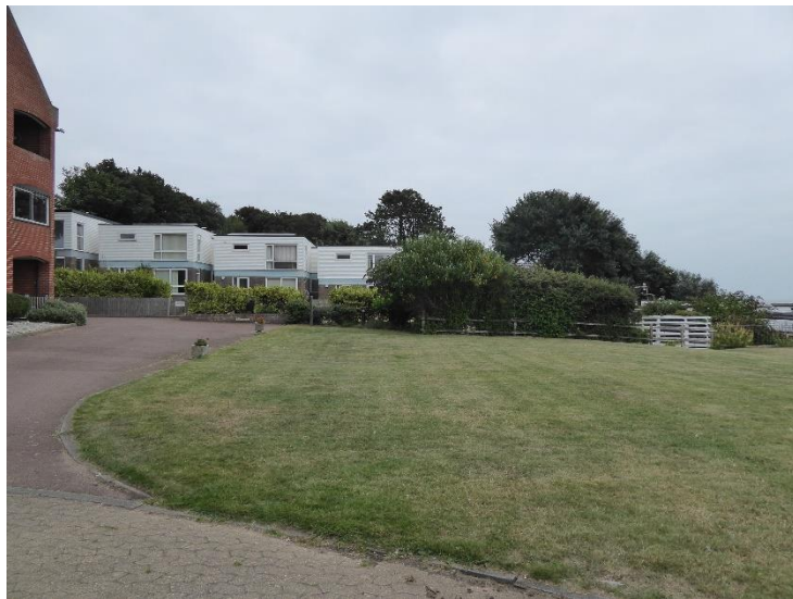
Figure 4 View north towards the row of staggered terraces
