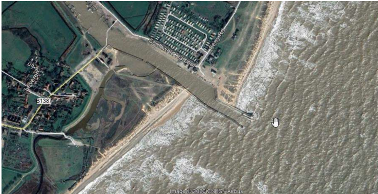
Figure 1-1 – Satellite image showing wave diffraction around the piers, and wave disturbance in the harbour entrance channel (Google Earth, 2020)
