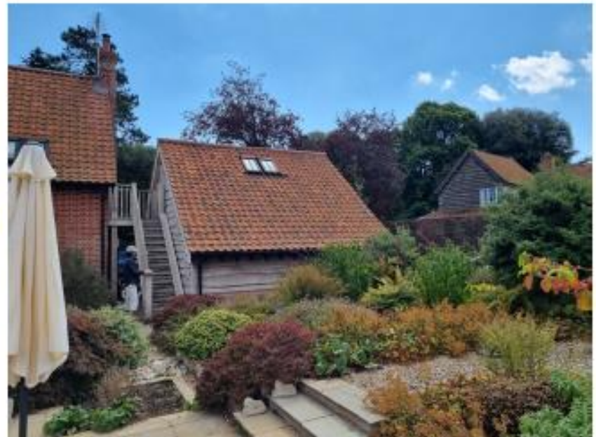
Existing cartlodge rear west elevation
