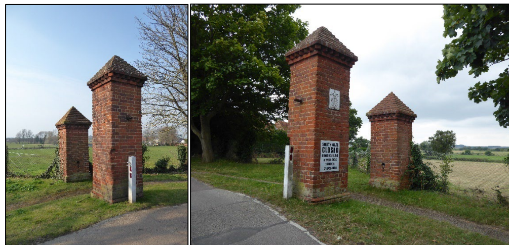
Figure 28: Gate piers at the northern entrance to the Conservation Area
