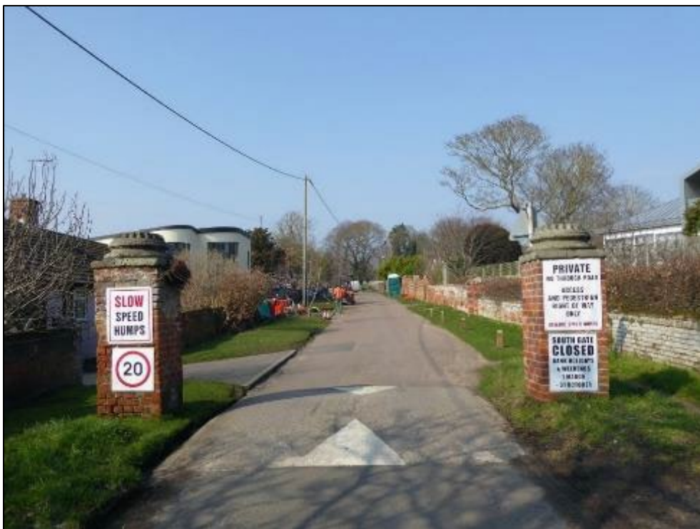
Figure 42: The Gate Piers at the southern entrance to the estate
