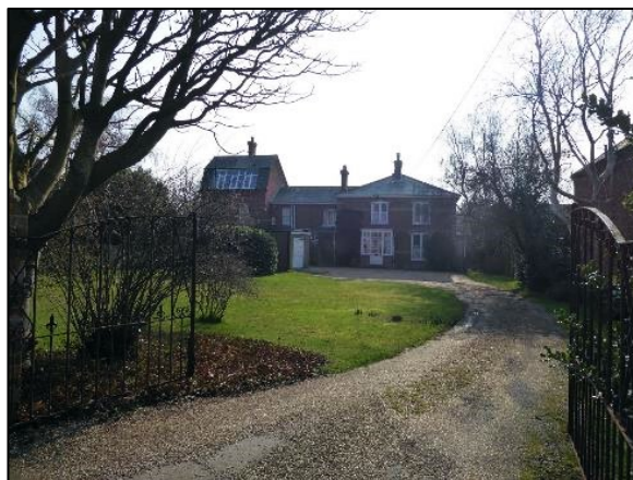
Figure 56: The Tower, Victoria Road
