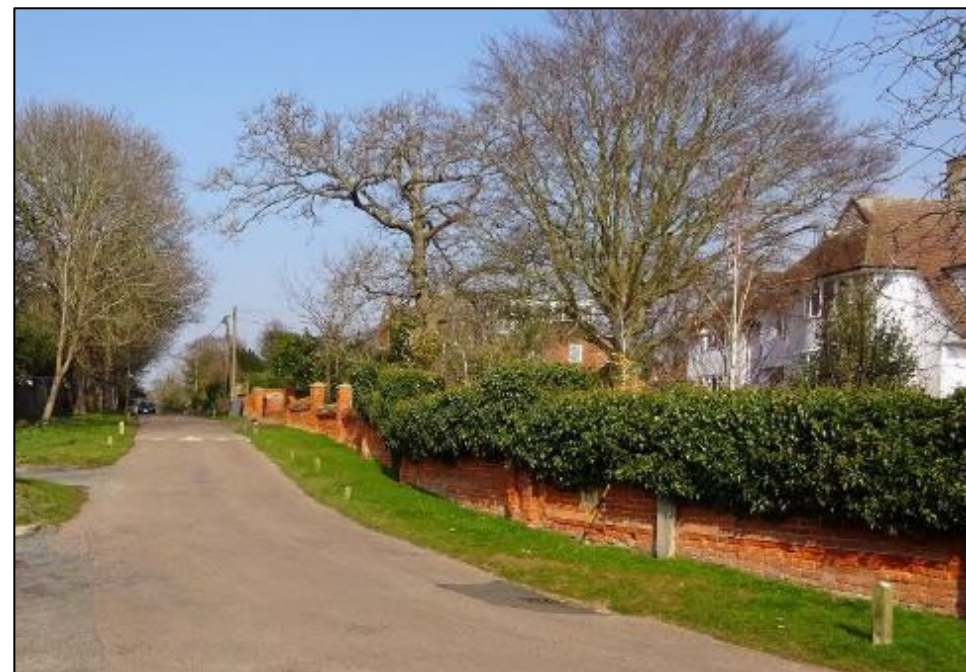
Figure 40: Original Wall and gate piers to 31 Park Road
