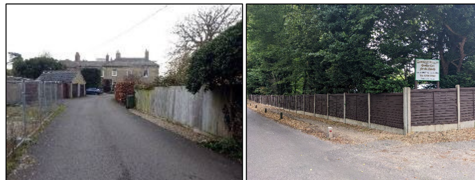
Figure 65: Examples of unsympathetic timber-boarded fences
