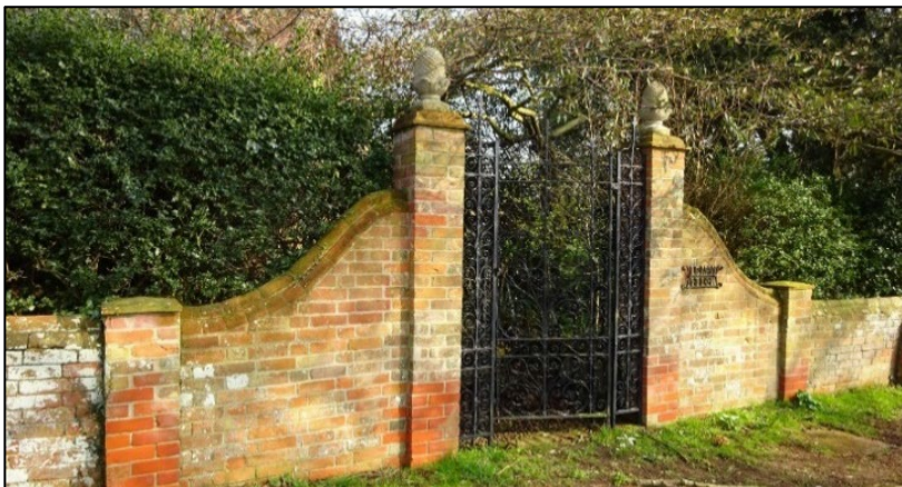
Figure 33: Boundary walls and iron gate leading to Dunan House
