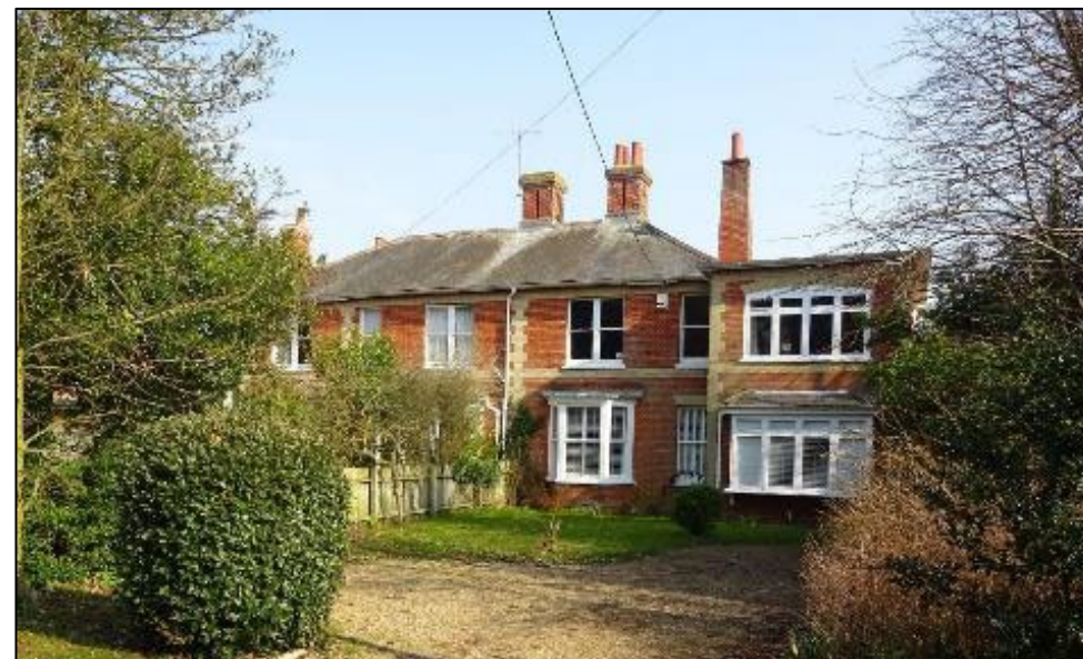
Figure 39: The Hollies and Hillcrest, Nos. 35 – 37 Park Road
