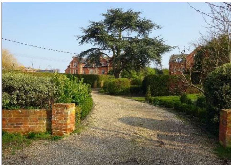
Figure 26: Belstead House (left) and No. 49 (right), Park Road
