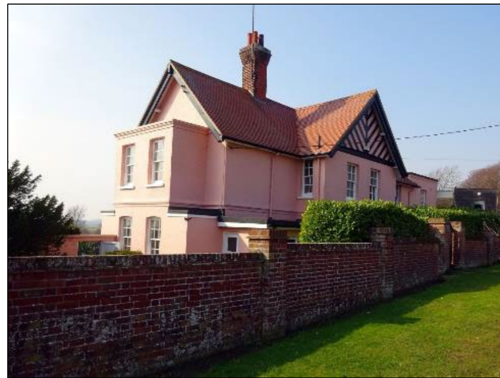
Figure 43: Park Lodge, No. 4 Park Road
