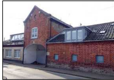
Figure 61: The original stable block to Alde House
