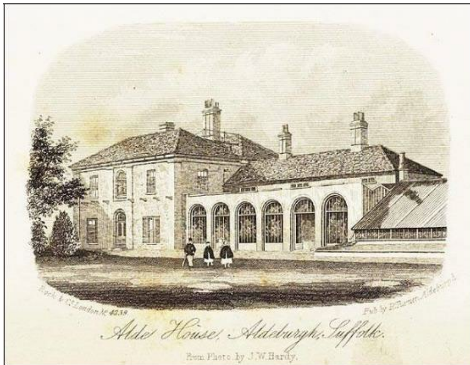
Figure 4: Alde House c1860
