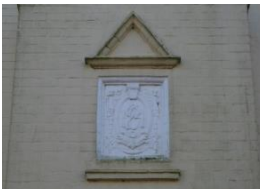
Figure 41 Date plaque on north elevation of No 4 Park Lane
