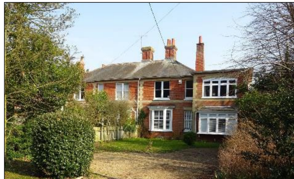
Figure 39: The Hollies and Hillcrest, Nos. 35 – 37 Park Road
