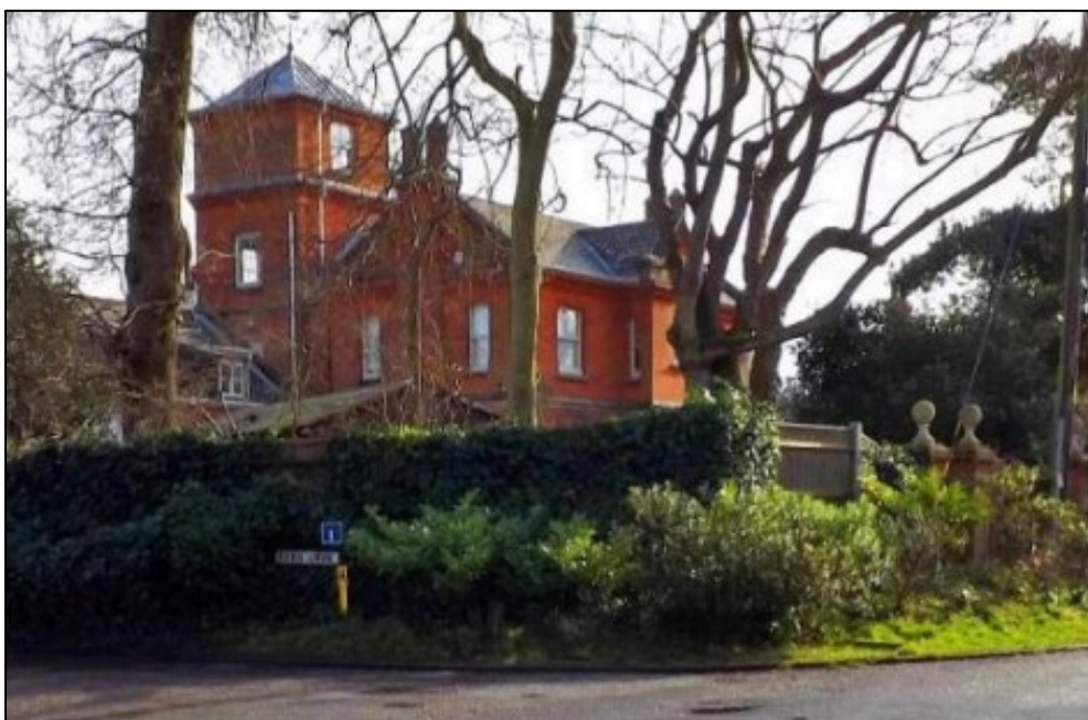
Figure 38: View of Fern Court from Park Road
