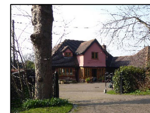
Figure 30: Modern property on Park Road
