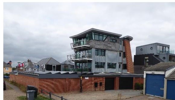
Figure 77 Latymer House, Brudenell Street
