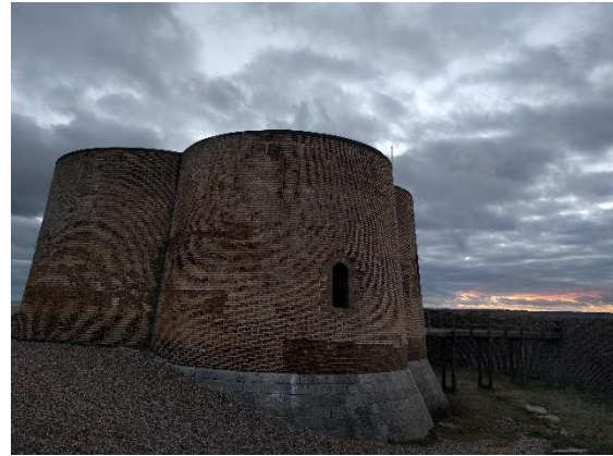
Figure 71 Martello Tower, Grade II*, List Entry Number: 1269724 from south
