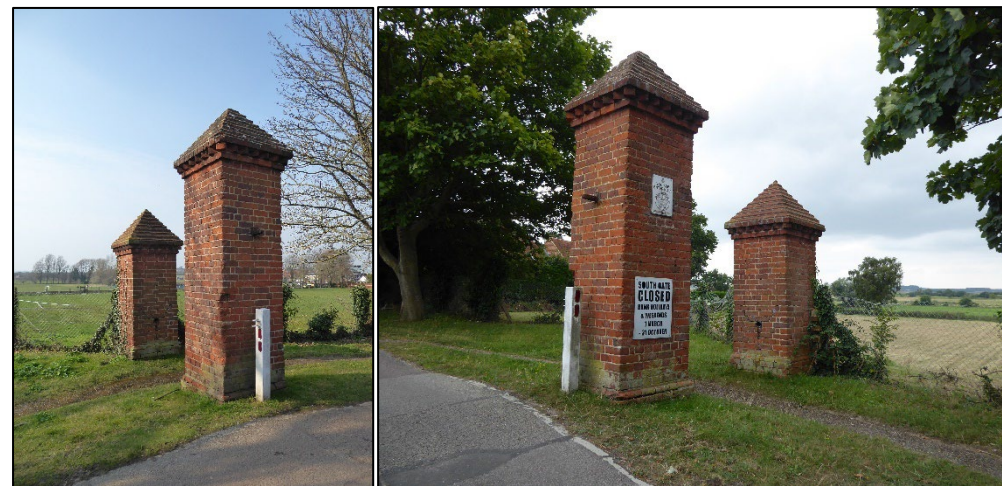
Figure 28: Gate piers at the northern entrance to the Conservation Area
