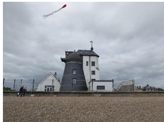
Figure 74 Old Mill House from the east
