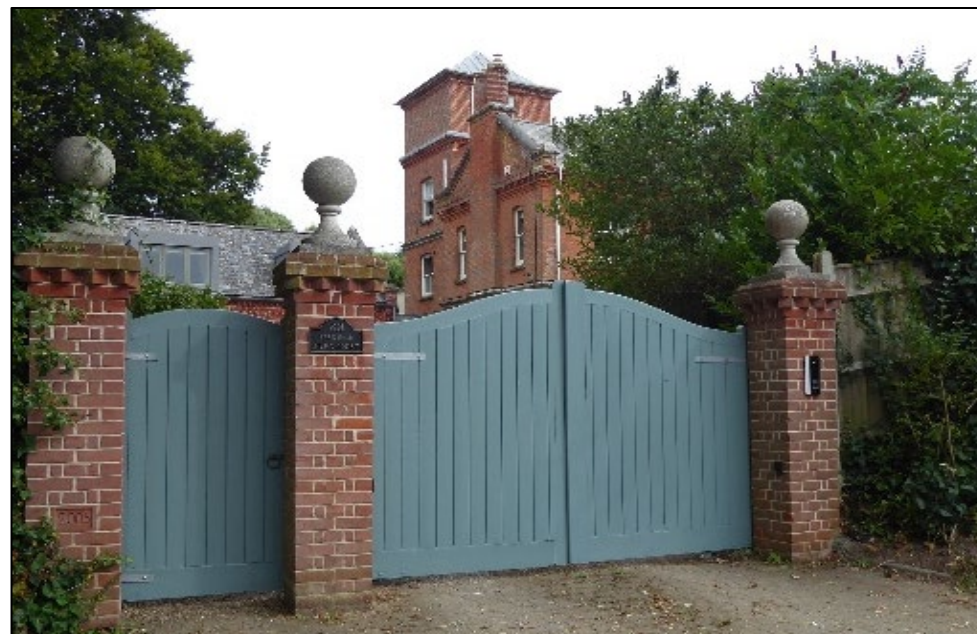
Figure 37: Fern Court behind red brick gate piers, topped with spherical finials
