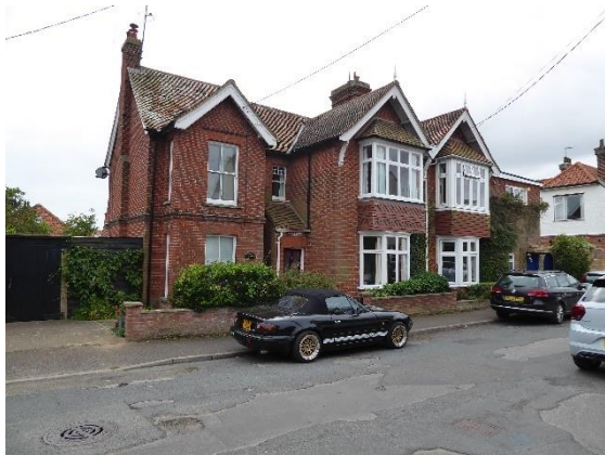
Figure 30 Nos. 8 - 9 Beaconsfield Road
