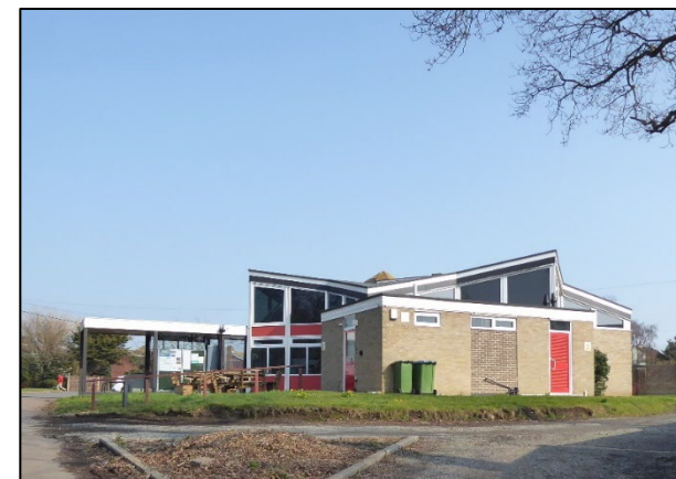
Figure 25: Aldeburgh Library, with prominent, angular roofline and porch extending to the left
