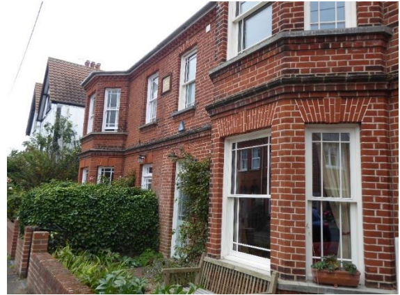
Figure 22 Example of red brick villa with bays, sashed windows, decorative banding, and dog toothed eaves detailing
