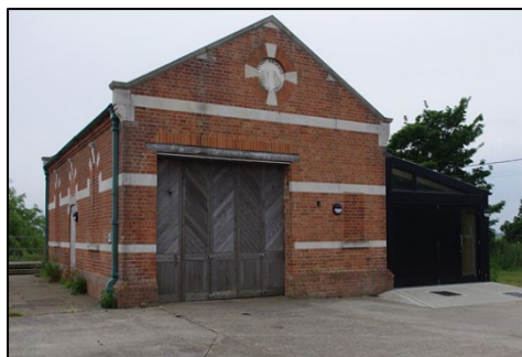
Figure 45: Sewerage Pumping Station
