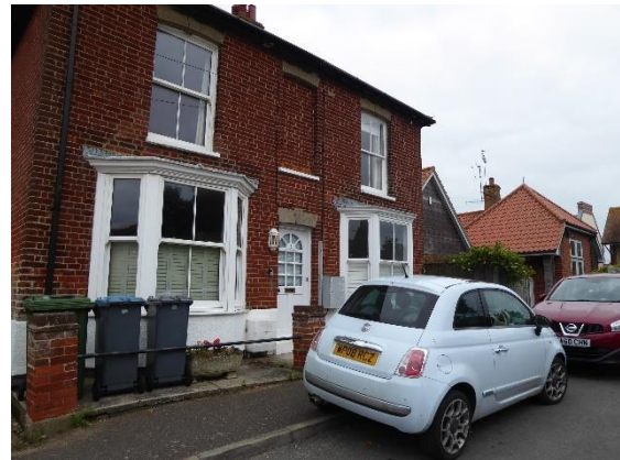
Figure 31 No. 5 Hartington Road
