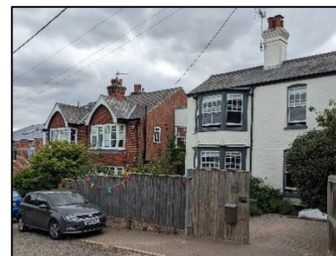
Figure 63: Nos 3 - 7 Crescent Road
