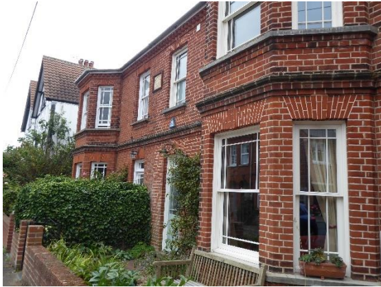
Figure 35 Nos. 9 - 11 Fawcett Road
