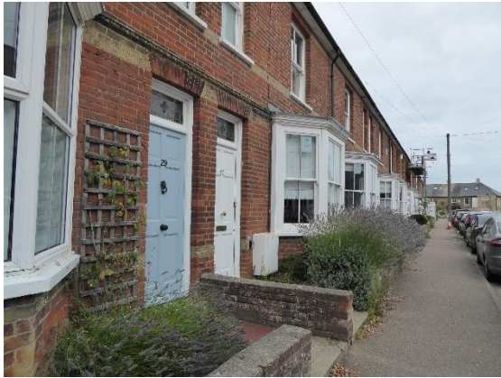
Figure 40 View north east along Park Lane
