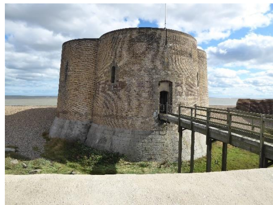
Figure 72 Martello Tower with the sea behind
