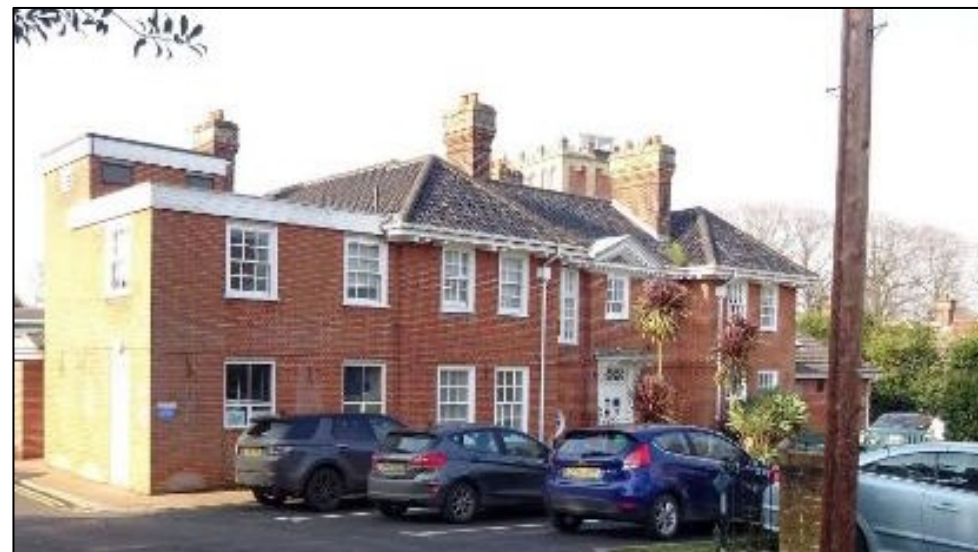
Figure 35: Aldeburgh Community Hospital (originally Dumfries)
