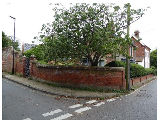
Figure 58 Historic walls on Crespigny Road
