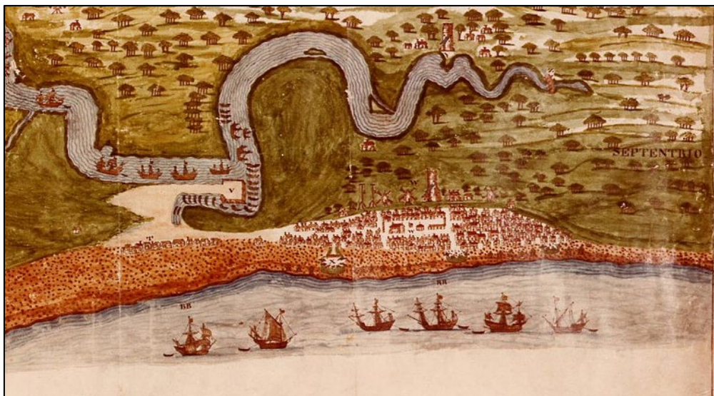
Figure 12: 1588 map showing Aldeburgh's historic town on the coastline, with the undeveloped marshland above, scattered with windmills
