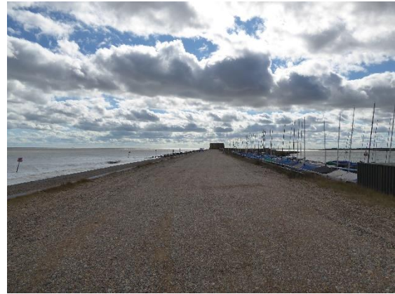
Figure 70 View south along the track towards the Martello Tower, with the Yacht Club to the right and shingle beach to the left, the openness of the area evident in the long view
