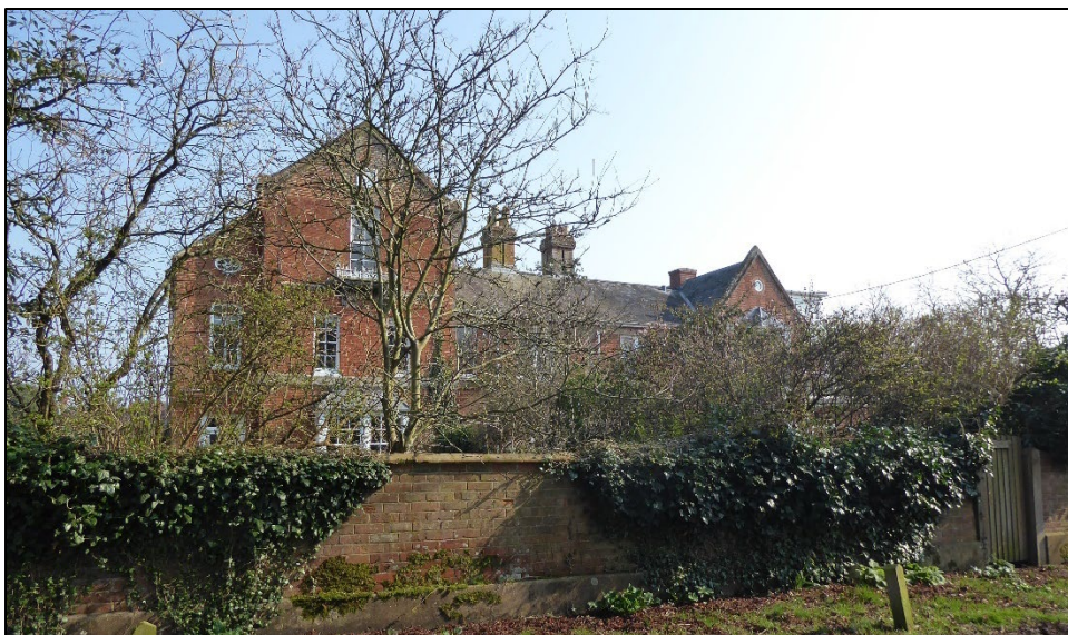
Figure 41: South House, Park Road
