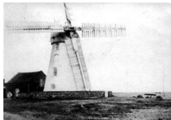
Figure 68 Fort Green Mill pre-1902 (source: Wikimedia commons)
