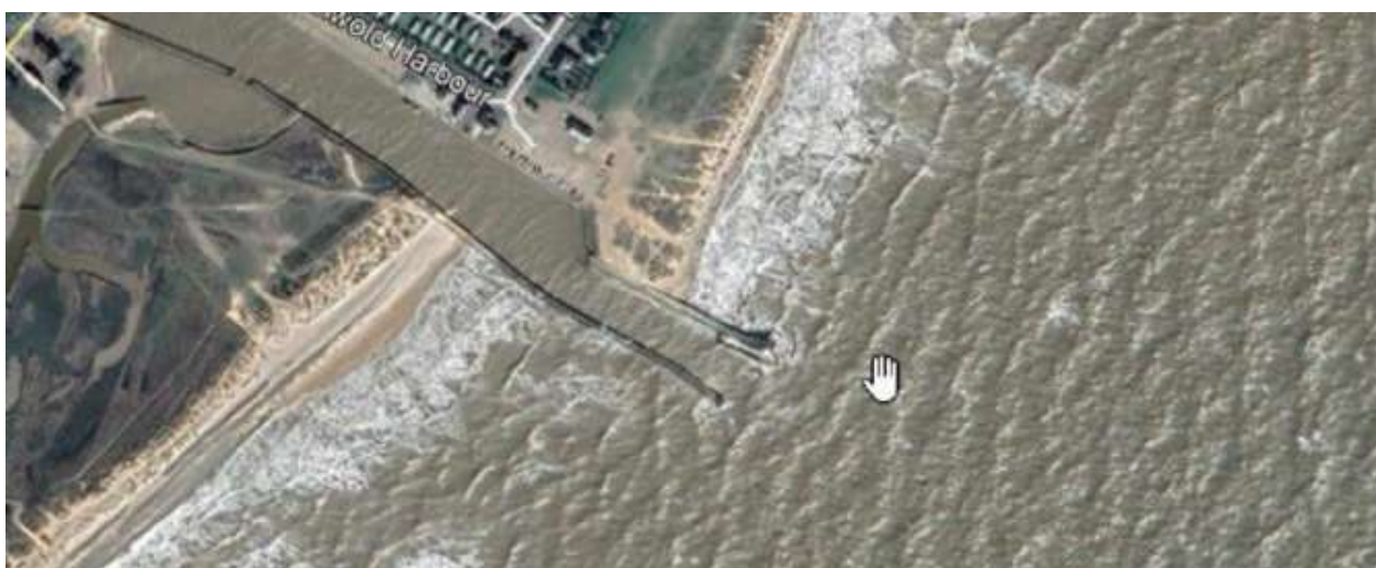
Figure 1-1: Satellite image - wave diffraction around the piers and wave disturbance in the entrance channel (Google Earth, 2020)
