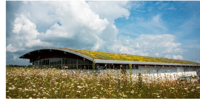
Green roof on the Adnams Distribution Centre, Reydon.
