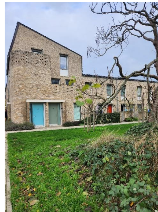
The Passivhaus homes in the Goldsmith Street development in Norwich are lower cost to heat, provide more consistent internal temperatures, are better ventilated, and are better sound insulated than homes built to Building Regulations minimums. Co-locating front doors also promotes neighbourly interactions.
