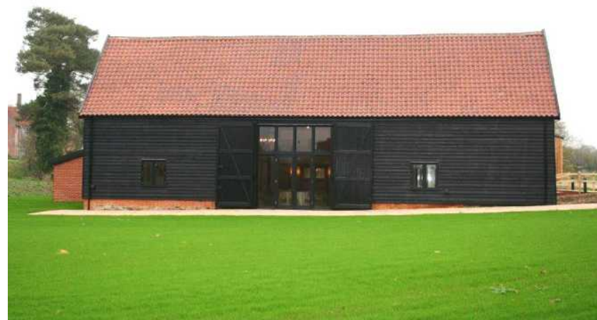
Converted barn with a limited number of openings in the wall, Bruisyard Hall Barns wedding venue (Source: Clive Tanner FRICS, Hollins Architects, Surveyors & Planning Consultants)
