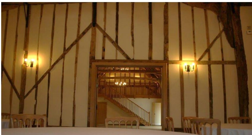
Converted barn with exposed timber stud walls retained, Bruisyard Hall Barns wedding venue (Source: Clive Tanner FRICS, Hollins Architects, Surveyors & Planning consultants)
