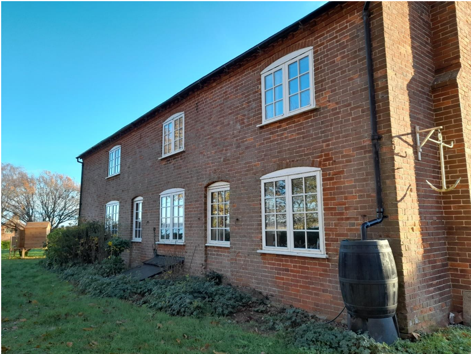
Existing north elevation – fronting the river
