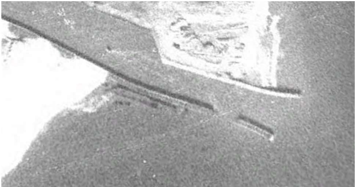
Figure 5 - 1945 aerial photo of damage to South Pier
