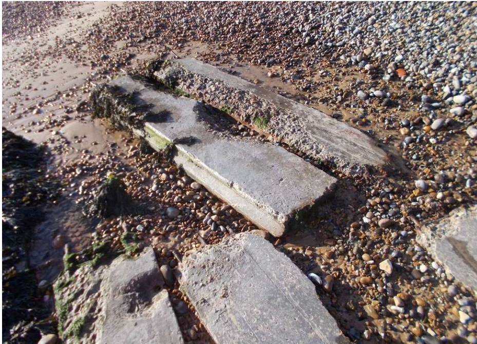
Figure 18 – Remains of upper lengths of cut planks from South Training Wall
