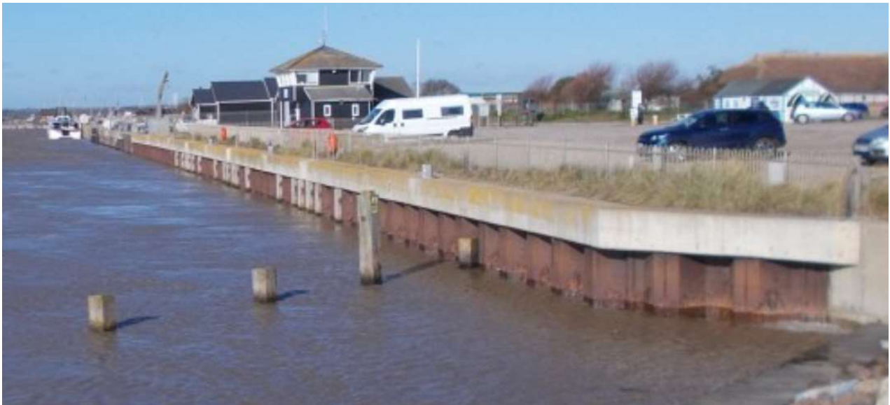
Figure 22 - Current condition of North Wall
