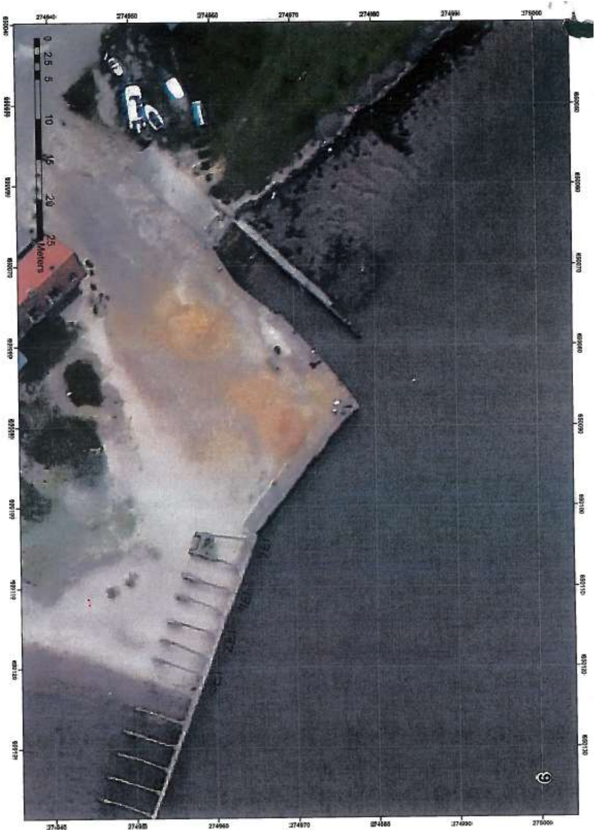
Figure A08 South Training wall and Slipway
