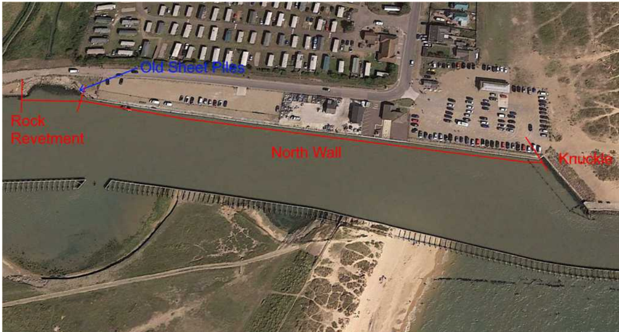
Figure 21 - Map of North Wall and rock revetment with old sheet piles marked
