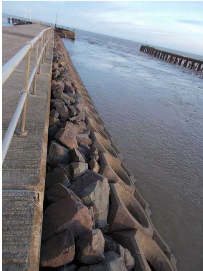
Figure 32 - SHED concrete blocks with rock fill
