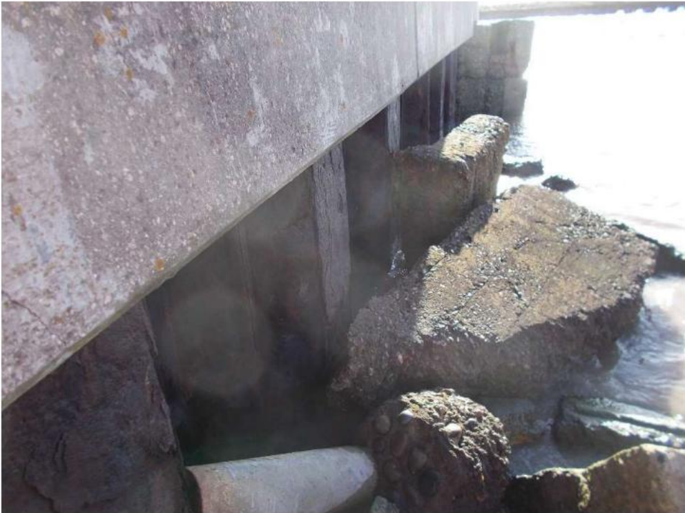
Figure 23 - Old Steel Sheet Piles at western end of North Wall
