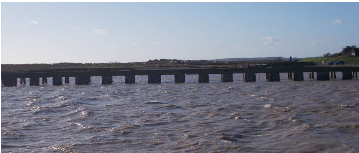
Figure 13 - Length of wall with windows cut in planks
