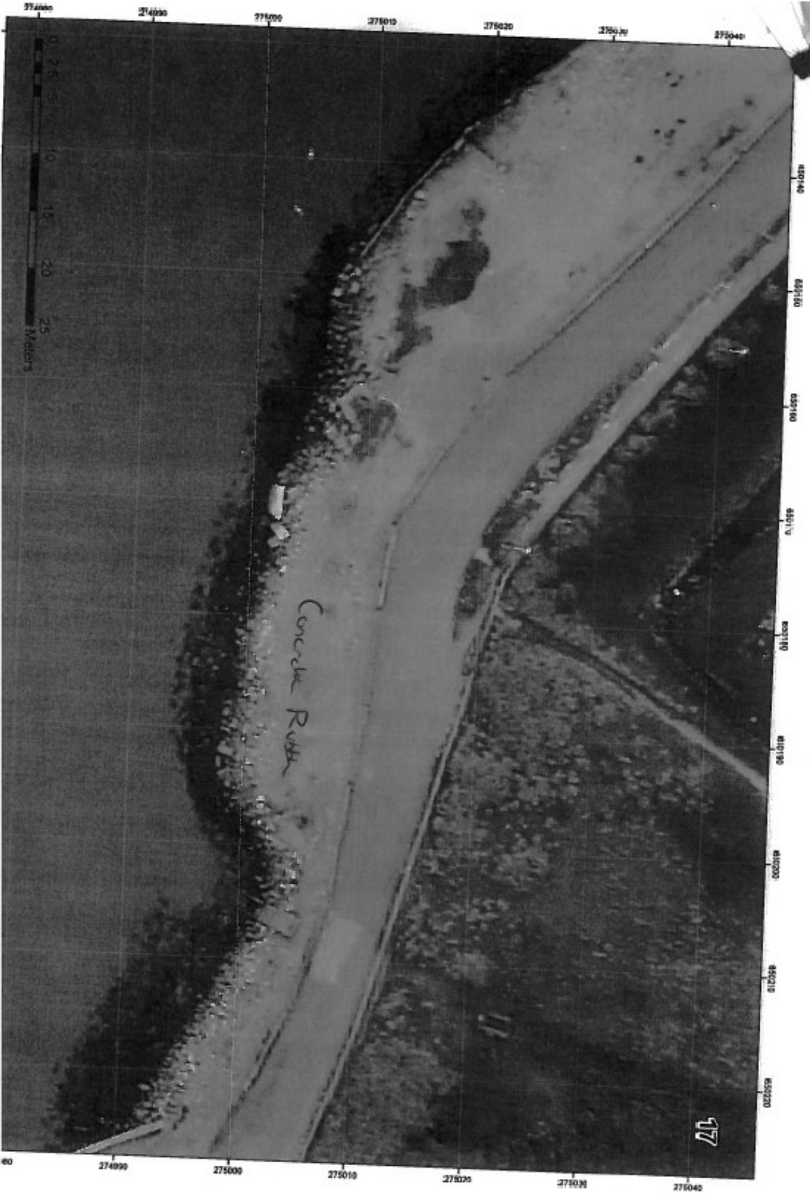
Figure A16 Rock revetment West of North Wall
