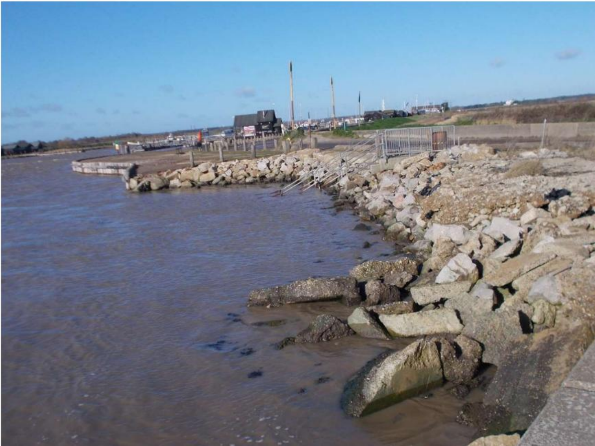
Figure 24 - Rock revetment West of North Wall
