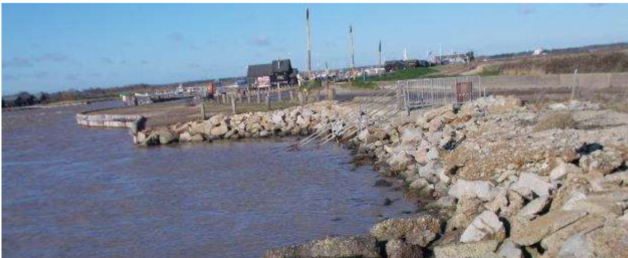
Figure 4-19: Rock revetment West of North Wall
