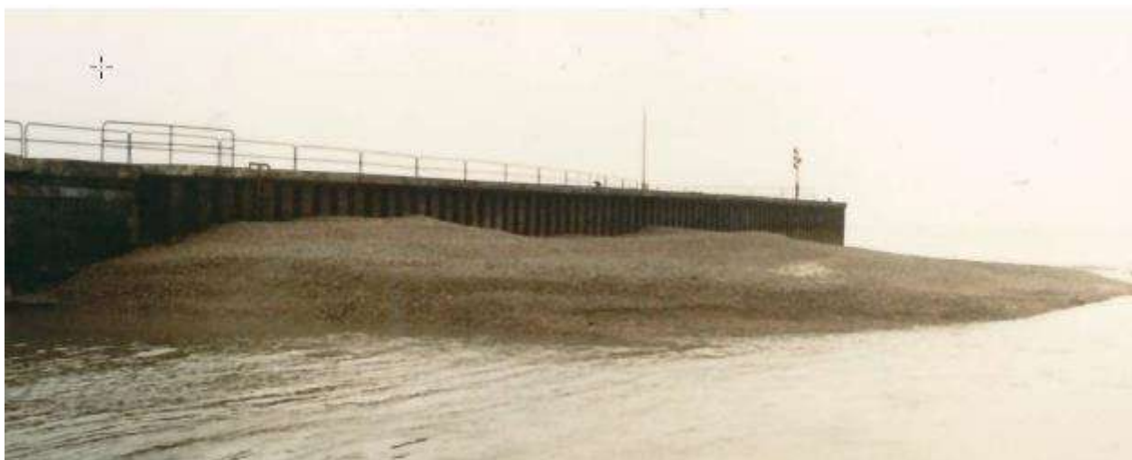
Figure 2-7: Sediment accumulation, north side of harbour, 1987
