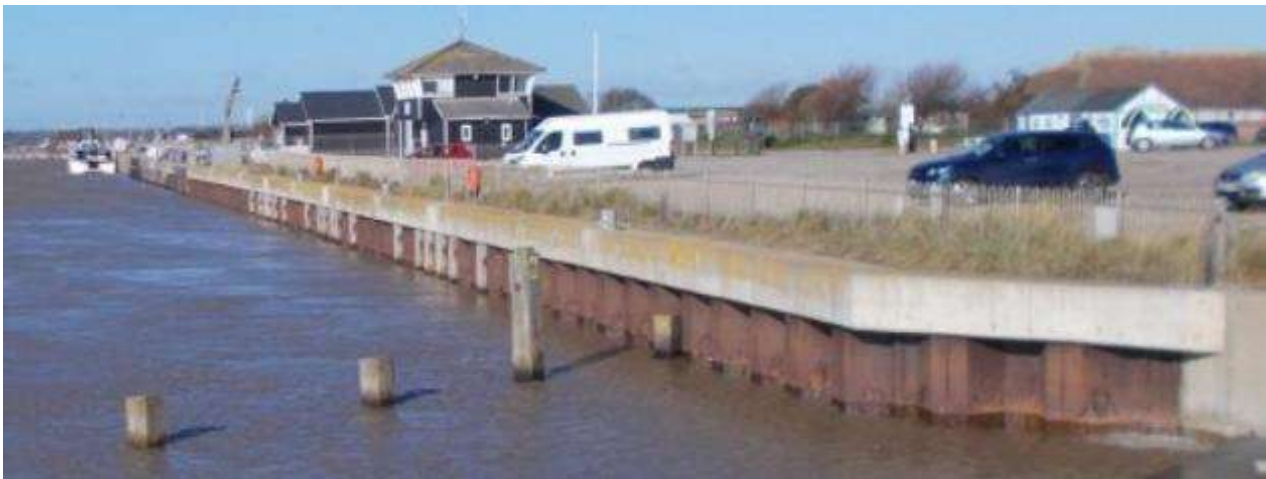
Figure 4-18: Current condition of North Wall
