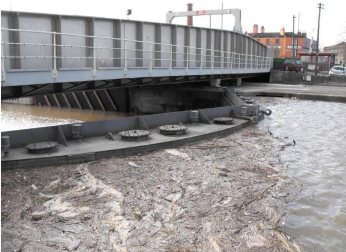
Plate 3-7: Mitre gates deployed against high surge.
