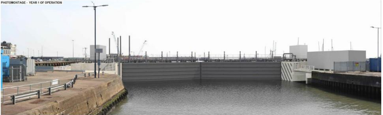
Plate 2-3: The proposed tidal barrier in the gate closed position (view looking east/seaward).
