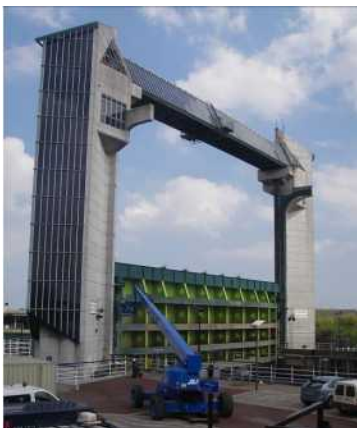
Plate 3-5: Up and over surge gate in Hull.
