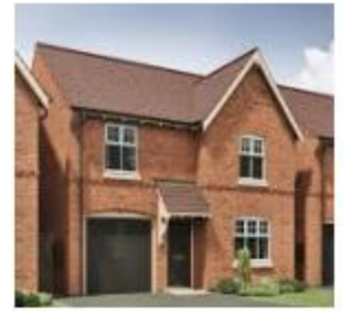
Gable Fronted Roof
