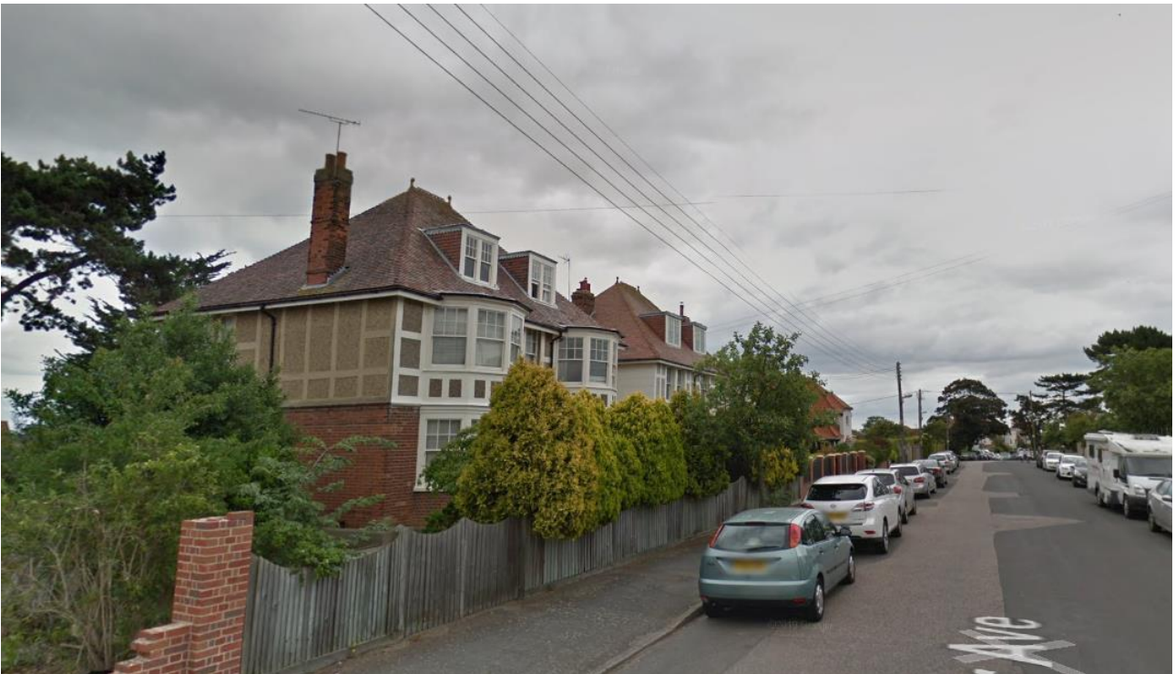
Figure 2 Pair of Edwardian villas on the opposite side of the street
