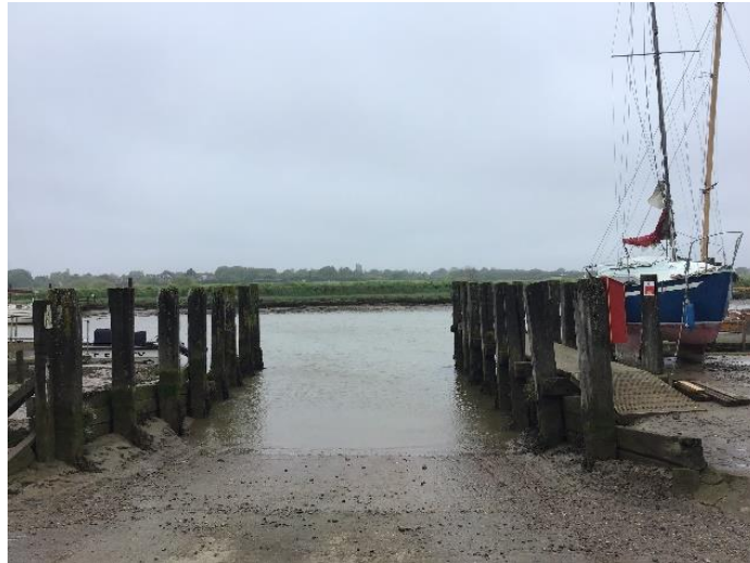
Figure 19 Slipway along the quayside
