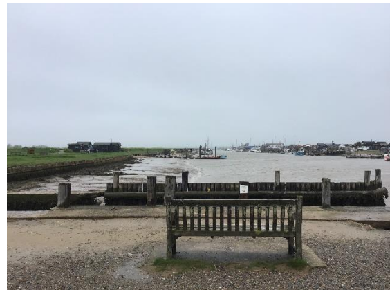
Figure 39 View north west along the River Blyth
