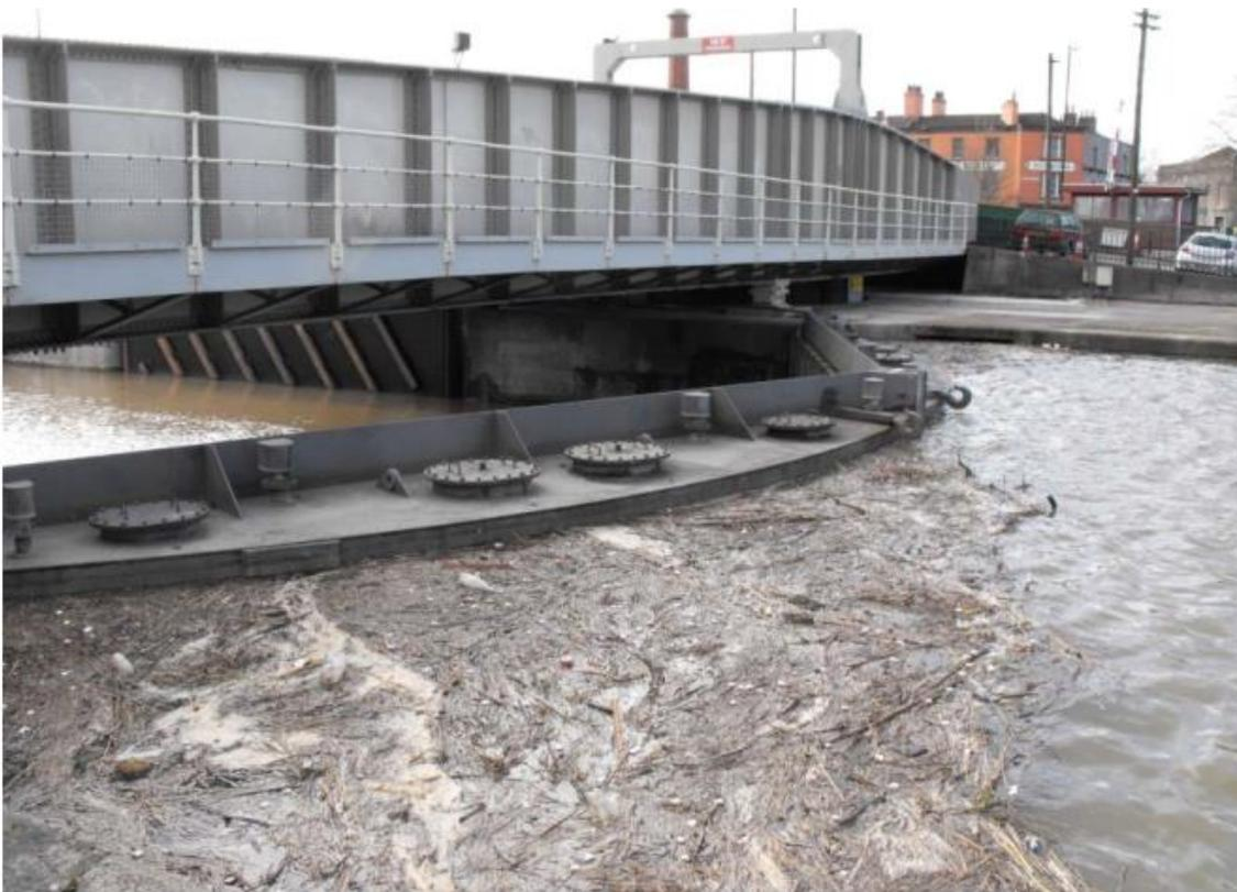
Plate 3-7: Mitre gates deployed against high surge.
