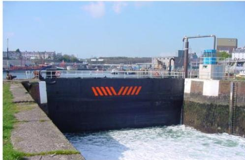
Plate 3-1: Side hinged caisson gate at Bristol.
