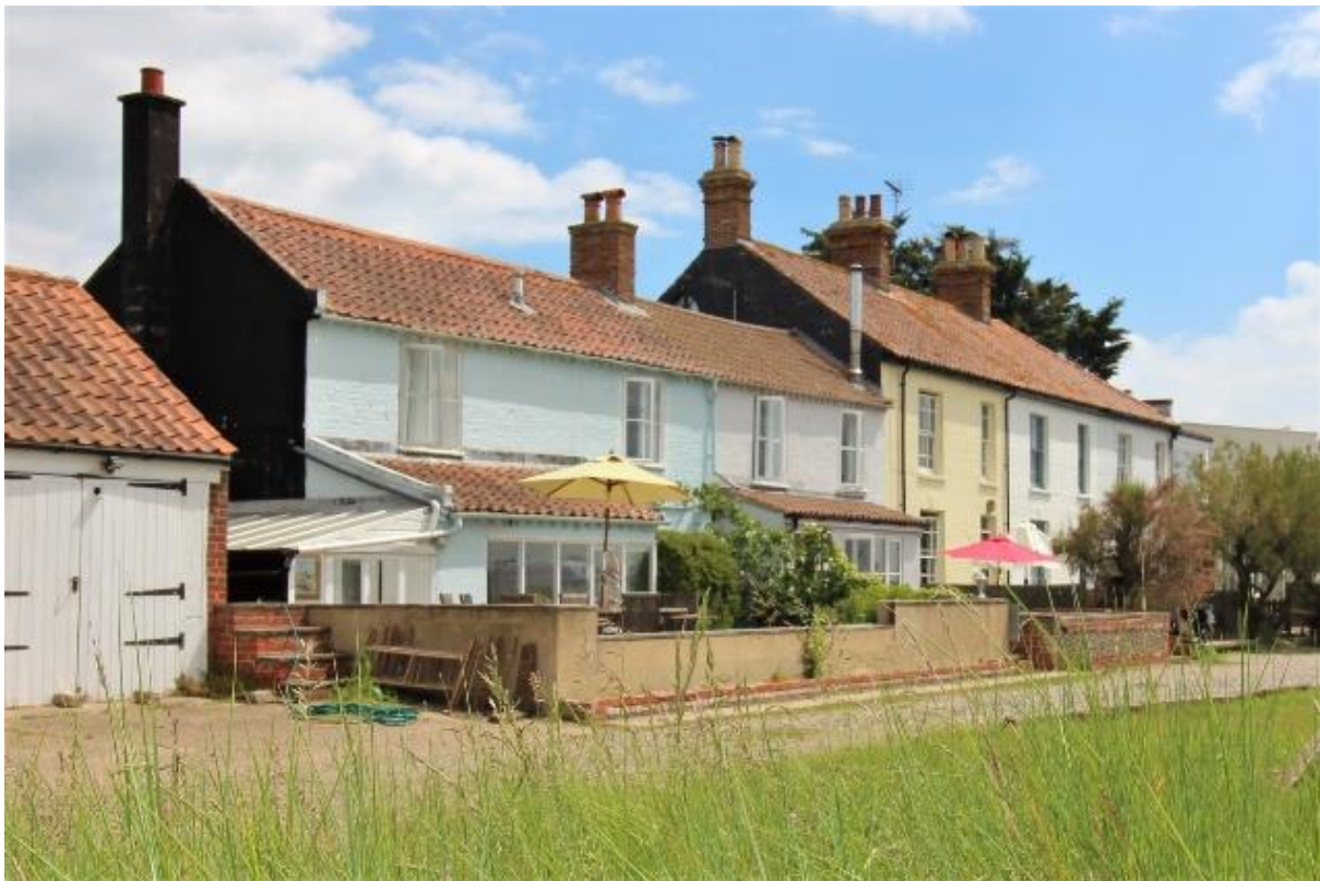
Blackshore Cottages from the southwest
