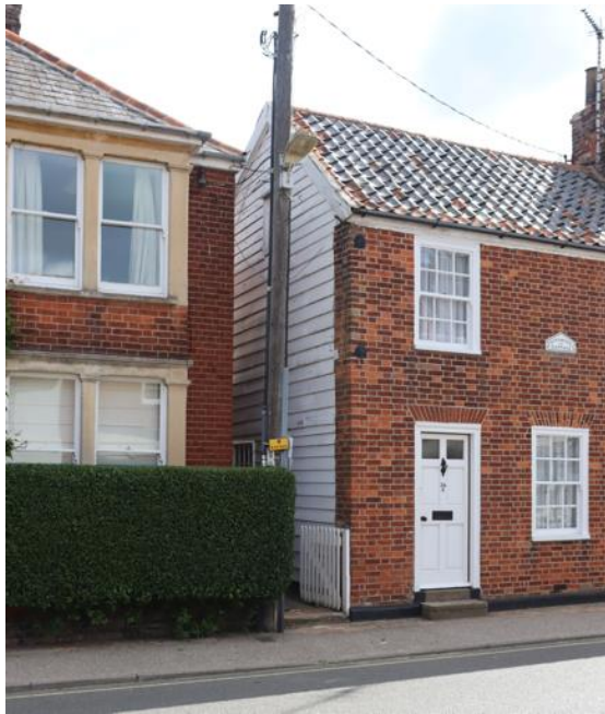
Weatherboarded side elevation to brick fronted cottage on the High Street.
