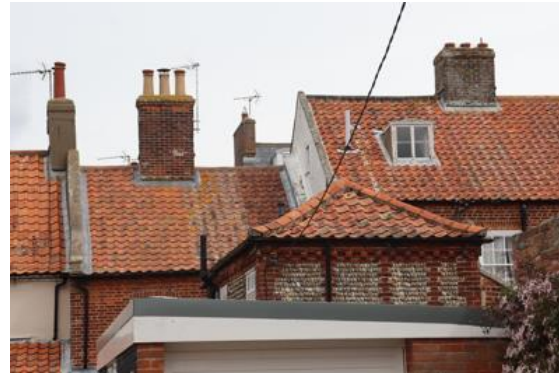
Red clay pan tile roof covering.
