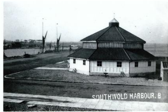
The Herring Processing Building known as the 'Kipperdrome', Ferry Road (demolished).
