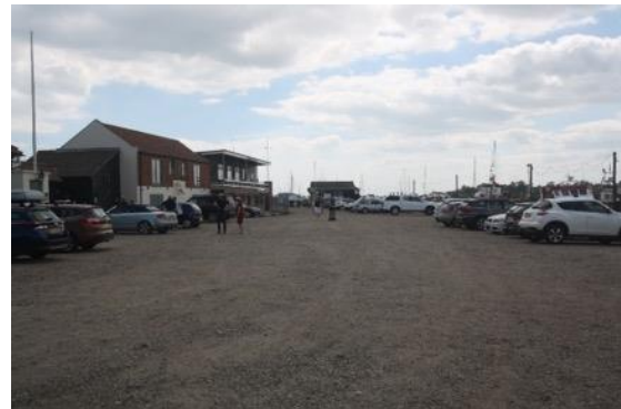
Access road at Southwold Harbour: like the built environment, the public realm is informal in character. Whilst this can lead to management issues, such as pot holing (below), the 'working' character of the public realm is equally important to the character area as the built environment.
