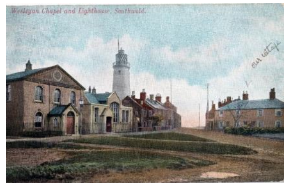
c.1900 Illustrated view east, over East Green and the surrounding informally finished roads; these have no kerbs or bitumen wearing course.
