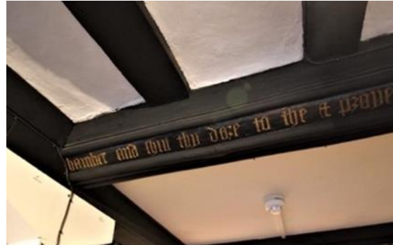
Re-used 16th century beam with inscription within commercial premises to the High Street.
