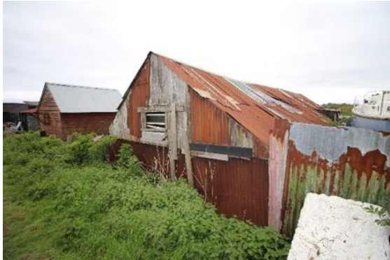
Former Boat Buildings Huts from the levee
