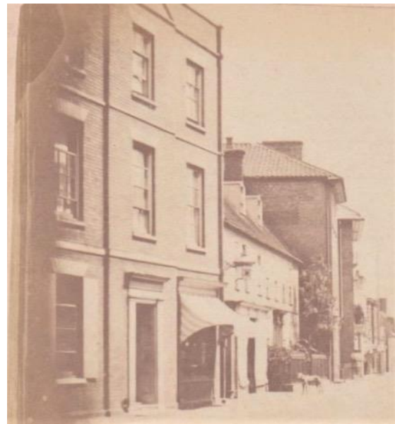
No.100 High Street, a purpose-built hotel of c.1834 built by the wealthy merchant James Robinson of No.17 Market Place to rival the nearby Swan, the townhouse beyond was destroyed by fire in the 1930s, from a carte de visite of c.1870.
