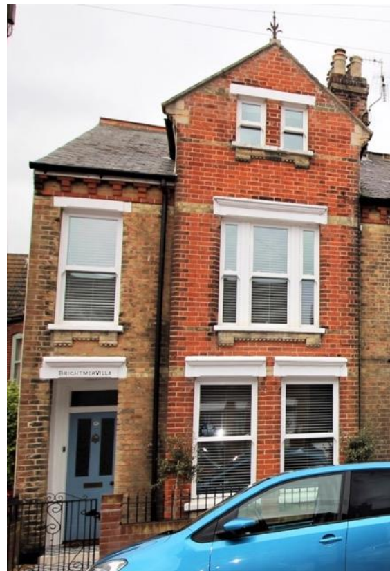
Brightmer Villa, Stradbroke Road a terrace displaying an inventive use of decorative brickwork.
