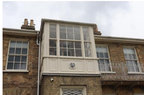
Timber square bay window.
