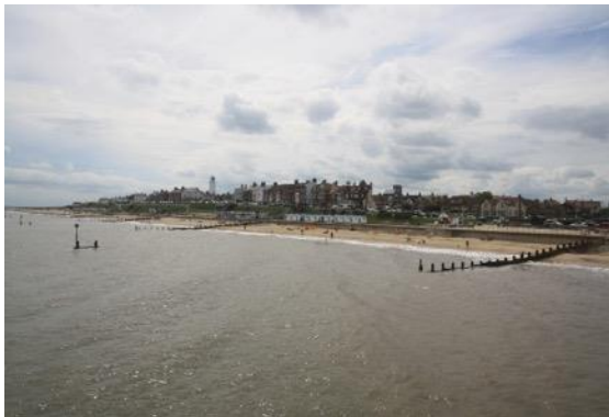
View of timber groynes, perpendicular to the coast and compartmentalising the beach to the south of the pier.
