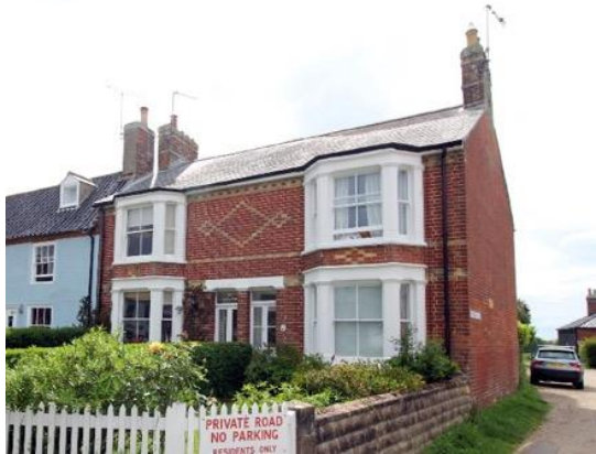
No. 14 Barnaby Green: Simple polychromatic brickwork enlivens the 19th century façade.
