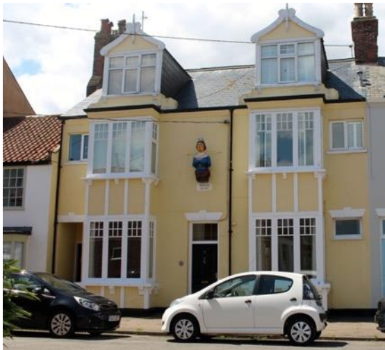
View of No.12 Stradbroke Road, Dolphin House and Douglas House, figure head on bracket above the front door.
