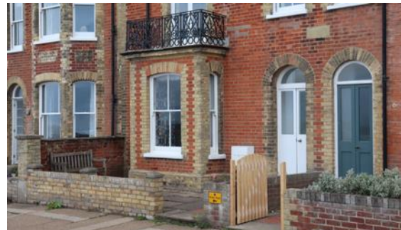
Plate glass sash windows, dating from the later 19 th century.
