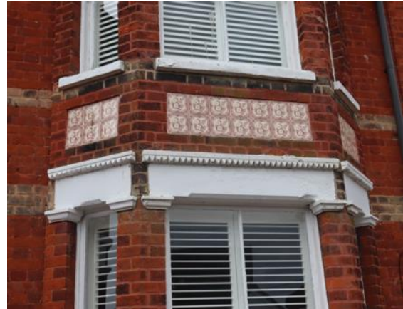
Inset Glazed Tile Detailing to the apron of bay windows.
