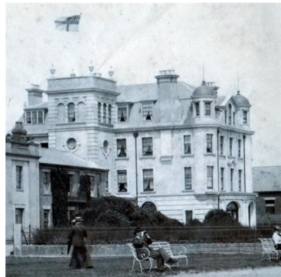
George Skipper's bedroom wing to The Centre Cliff Hotel of c.1905, its two upper floors have since sadly been removed.
