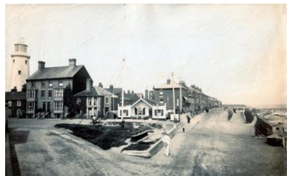
St James' Green: prior to cement render on earlier block wall and steps.
