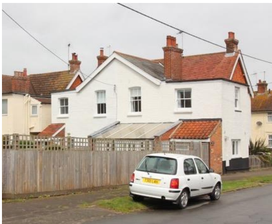
Rear of c.1905 houses on North Road from St Edmunds Road.
