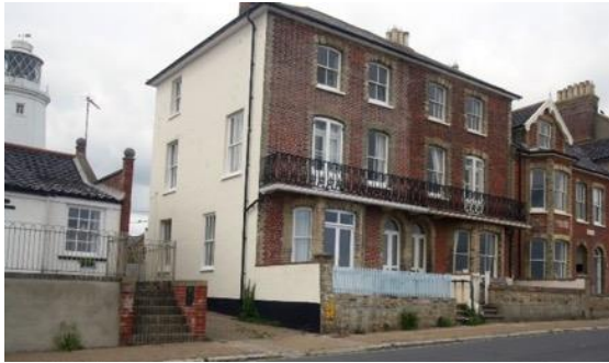
North Parade: decorative ironwork makes a positive contribution to the significance of the Conservation Area, however, the front boundary wall has been largely rebuilt with unremarkable timber fence above.
