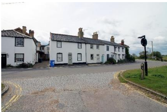
Constitution Hill: Small areas of granite setts as junction treatments.
