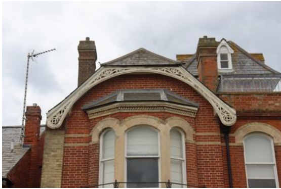
Slate roof covering.
