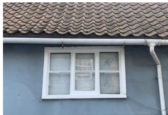
Timber casement window, possibly dating from the late 18 th century.
