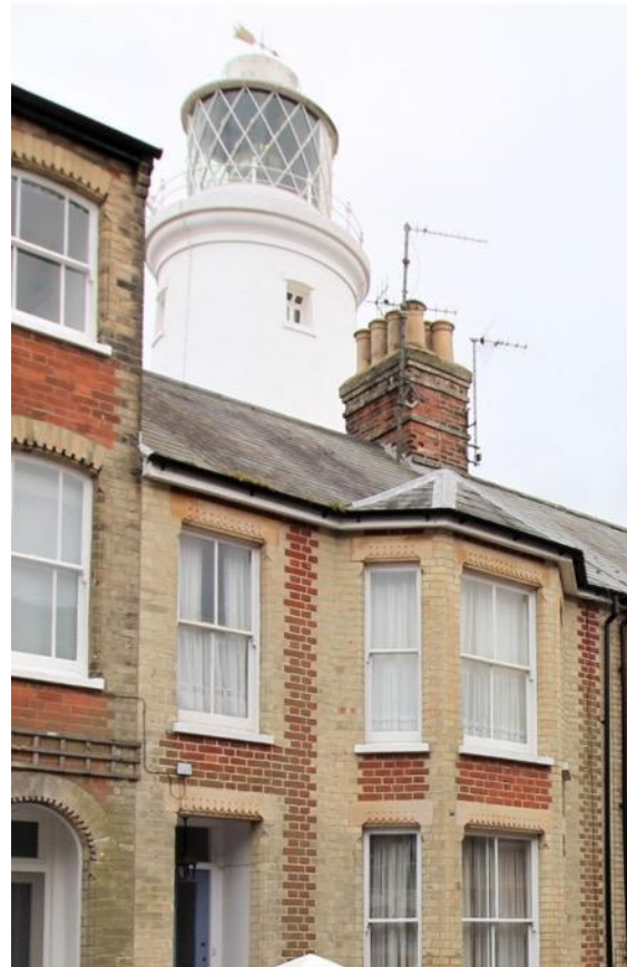
Chester Road: recently cleaned brick work.
