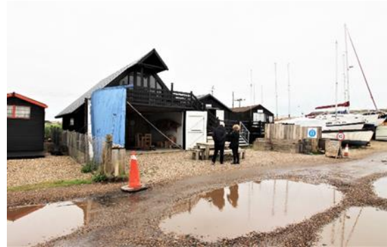
The assertively designed Novoboats Building a recent addition to the Blackshore huts.
