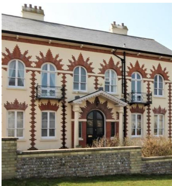
Suffolk red brick, used to ornament Southwold House & Sole Bay House, Gun Hill, in contrast to the render.
