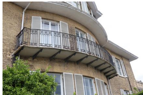
Elaborate wrought iron railings with curved ‘bombe’ base.
