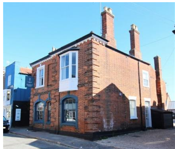
No.8 East Street: An externally well-preserved former public house that is now a shop.
