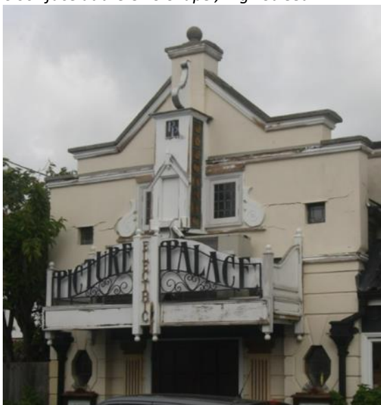
Elaborate signage at the Electric Picture Palace, Blackmill Road
