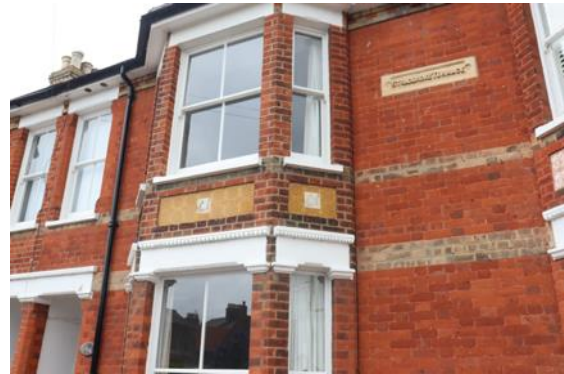
Detail of canted bay window with plate glass horned sash windows.
