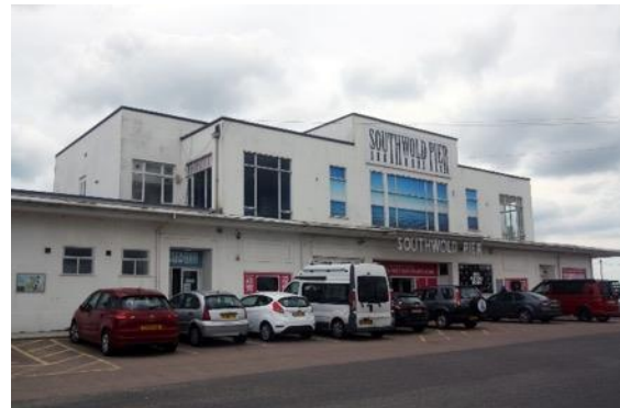
The bitumen car park setting of the pier head.
