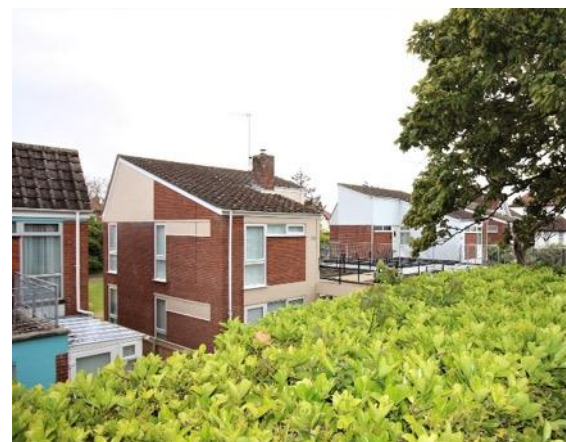
Inventively designed late 1960s housing Nos.72-78 (even) Pier Avenue
