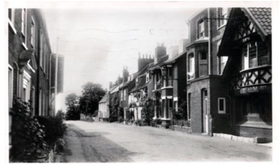
Park Lane, prior to highway alterations show the streets edge-to-edge carriageway and crushed stone material.
