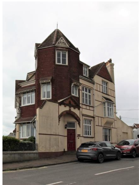
The Field Stile Road elevation of the c.1895 No.28 North Parade, this was designed to overlook the forecourt of the now demolished Grand Hotel.
