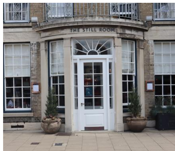
Curved bay window (central door is a later insertion).
