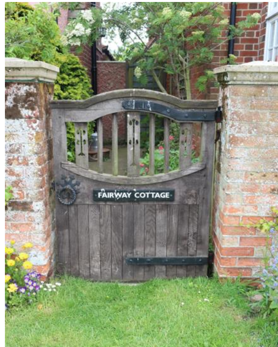
Timber hand gate with bespoke strap hinges and ring handle, designed to complement the timber screen.
