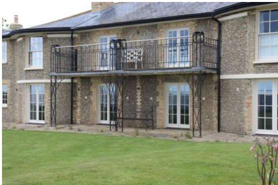
Restrained iron railings, supported below to form first floor balcony and covered ground floor veranda
