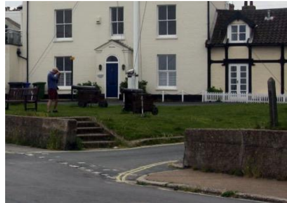
St James' Green: modern cement render (top) on earlier block wall and steps (below).
