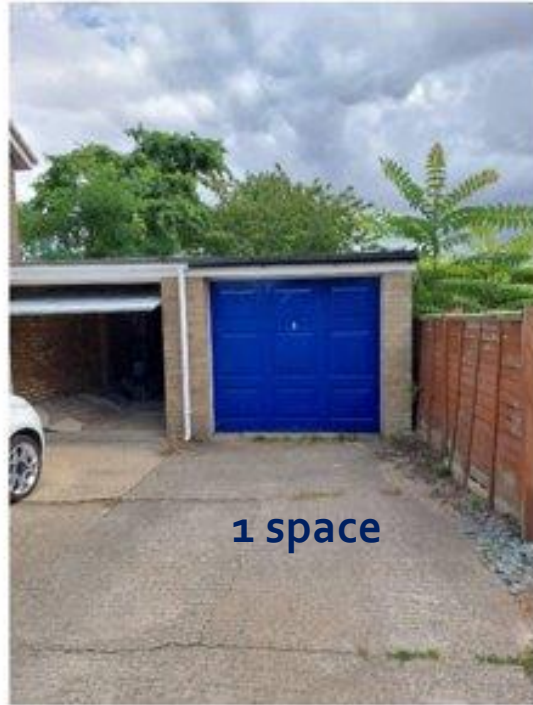
Front of existing garage
