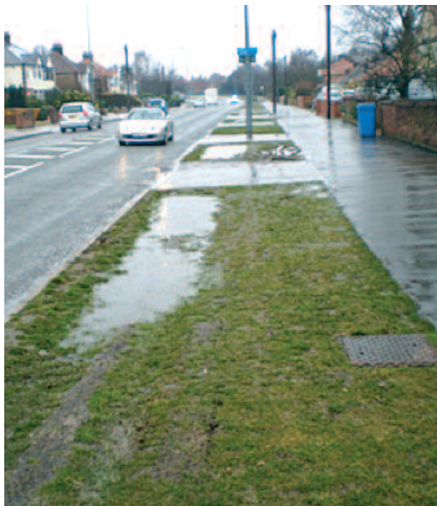
BEFORE: Newly completed Retrofit SuDS at Heath Rd, Ipswich. Shallow basins were rutted and damaged in wet weather by cars parking on new verges.
