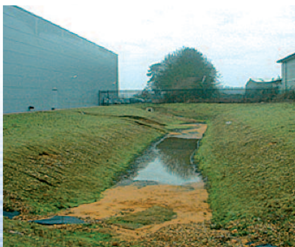
Poor inlet design causes erosion and deposition of sediment and a reduction in infiltration capacity.
