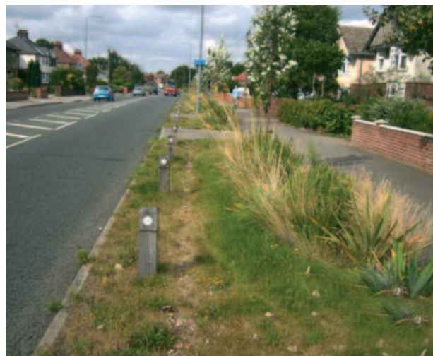
AFTER: Heath Road, Ipswich with deterrent posts and planting. Timber posts have been utilised on the carriageway side along with deterrent planting on the footway side. A small gravel trench was constructed to provide additional storage and soakage.
