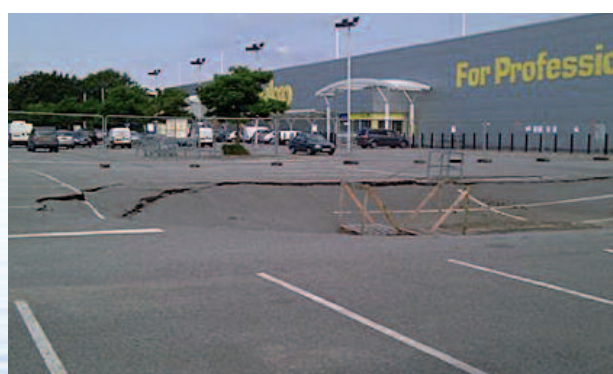
The failure of a plastic geocellular tank under a car park in August 2012. The cause of the failure is not currently known.
