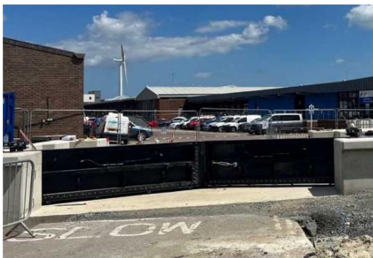
Flood gates installed in the port entrance.
