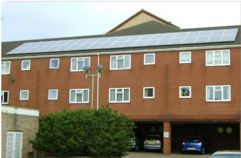
Example of a retired living scheme in East Suffolk where a south facing roof face provided an opportunity to install Solar PV panels to improve the energy efficiency of the building.
