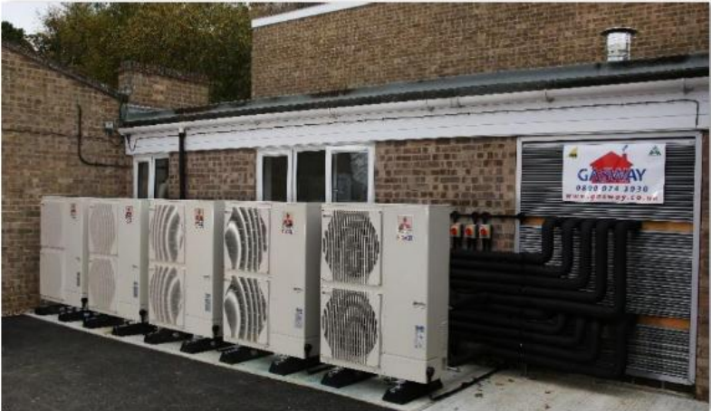
Example of a retired living scheme in East Suffolk that was fitted with a commercial air source heating system to improve the energy efficiency of the building.
