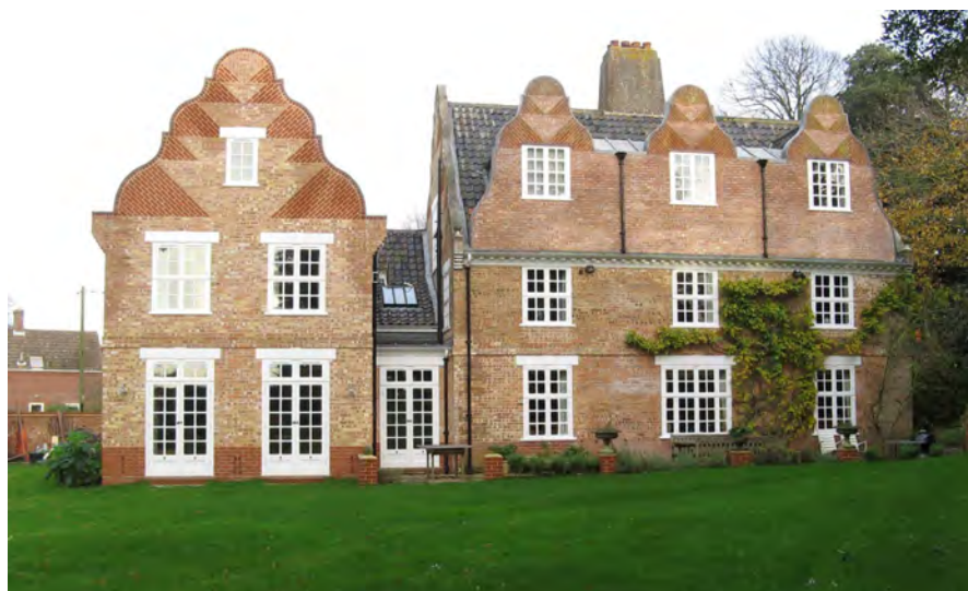
A successful extension (left of picture), which uses the same brick patterns and colours, as well as the same windows, as the original (Dolphin house, Aldeburgh). (Source – NJ Architects; photo by Andrew Hendry)
