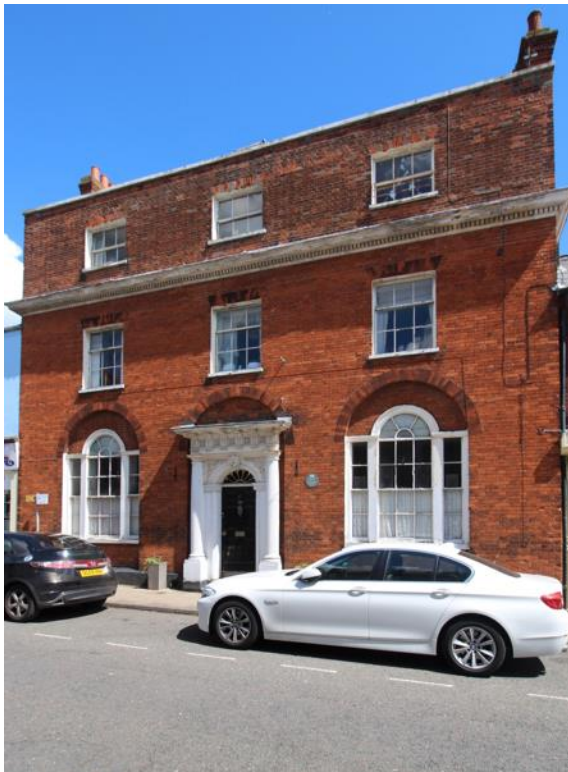
Red brick elevations with gauged brick arches
