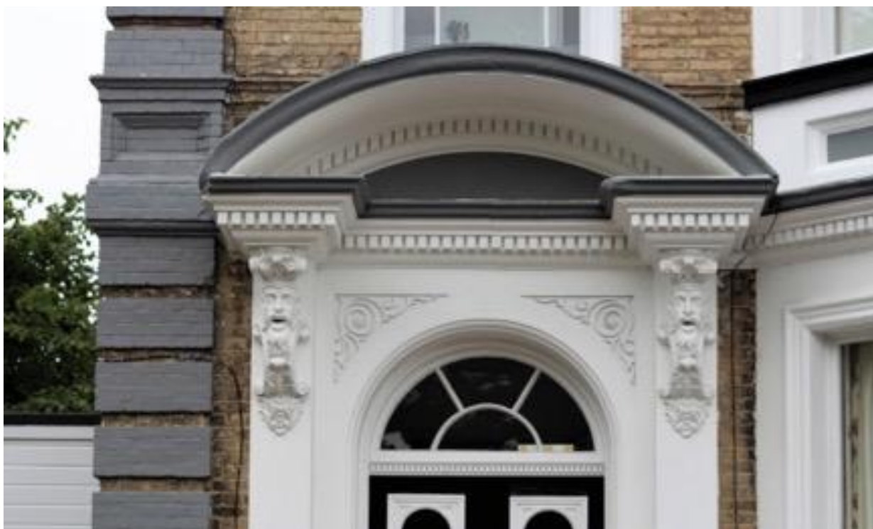
Finely Detailed Stone Door Surround with Dentilled Curved Pediment, North Parade
