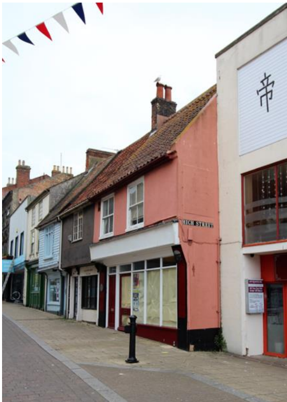
Painted render or stucco elevations
