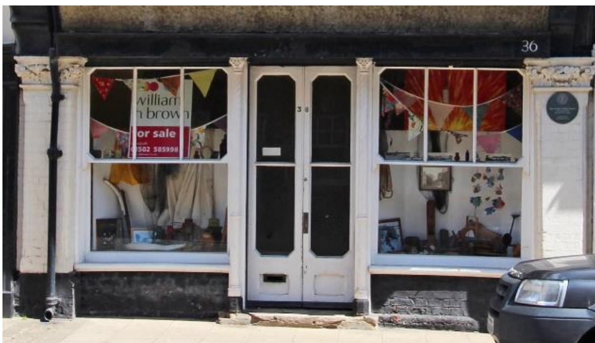
Detail of No.36 High Street. A late 19th-century shopfront with cast-iron columns set below the jetty of a 15 th century house
