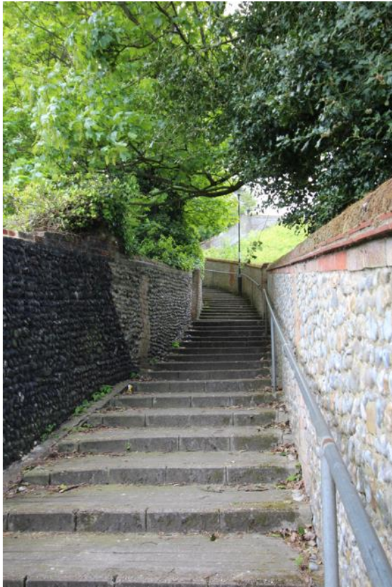
Cobble walls and stone nosing to steps
