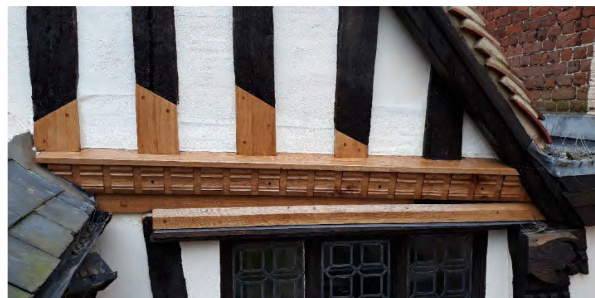
Before and After decayed timber repair (Source – Rick Lewis, Traditional Oak Carpentry Ltd)
