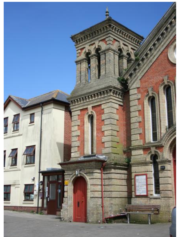
Red brick elevations with white brick dressings
