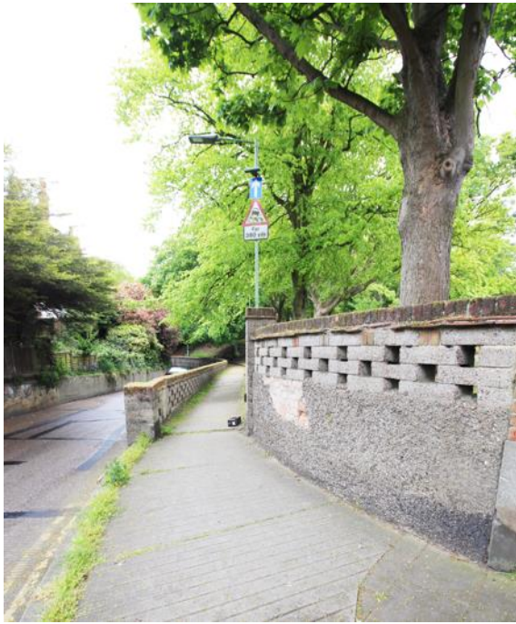
Cast concrete walls and balustrades
