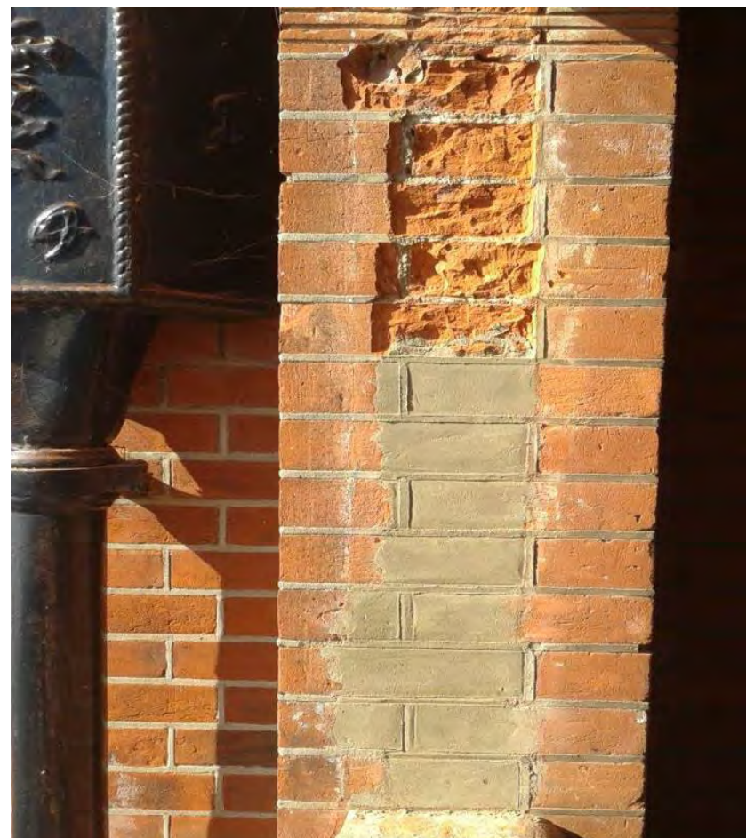
Broken brickwork prior to repair (The Bartlett Hospital, Felixstowe) (Source – Patrick Allen & Associates)
