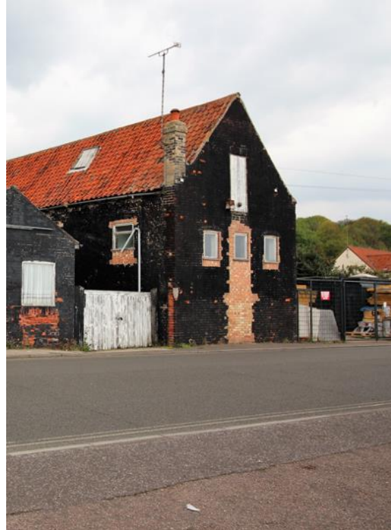
Black painted or tarred brickwork
