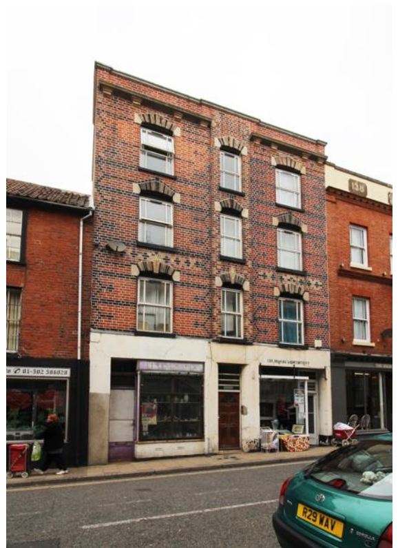
Polychromatic brickwork
