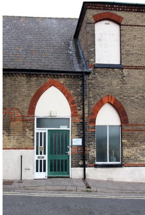
Poor quality replacement joinery, Herring Fishery Score
