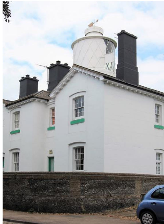
Rendered elevations with ashlar marking
