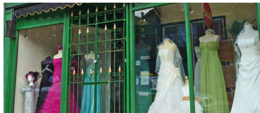
A traditional grille protecting the entrance to a shopfront (Lowestoft)
