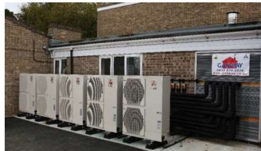
Figure 6 Air Source Heat Pump System
