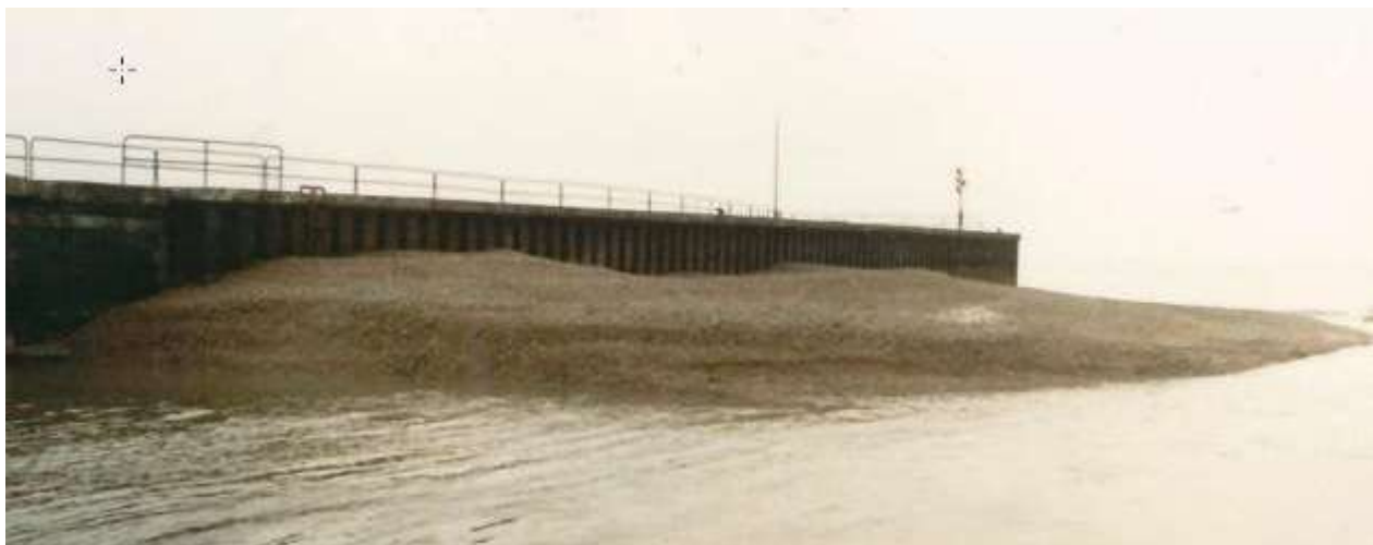
Figure 3-1: Sediment accumulation, north side of harbour, 1987
