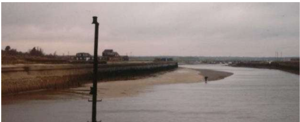
Figure 3-2: Sediment accumulation, south side of harbour, 1987
