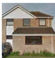
Combining materials - brick and cladding boarding
