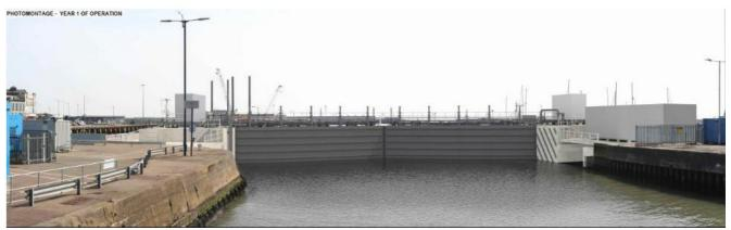
Plate 2-3: The proposed tidal barrier in the gate closed position (view looking east/seaward).
